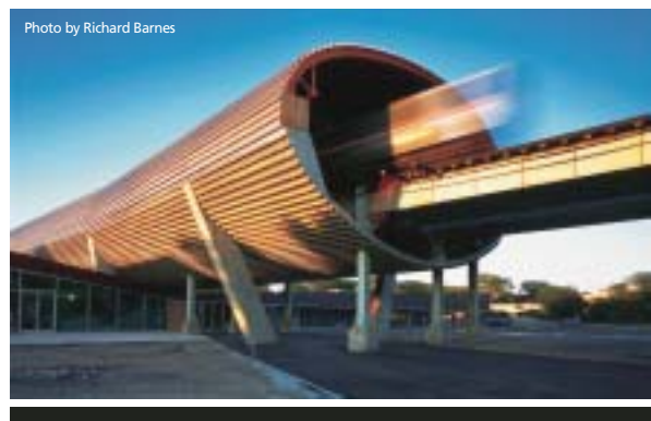
A soundproofing tube surrounds the Green Line track at the Illinois Institute of Technology.
