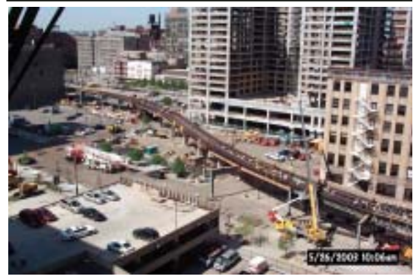
The curved track at Harrison Curve was removed and replaced with a new, more linear track. These before and after photos show what the CTA can accomplish in a weekend.
