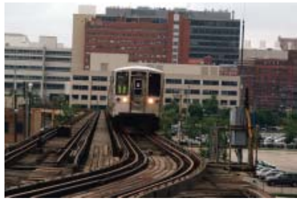
Renovation of the Paulina Connector will be completed in 2005.
