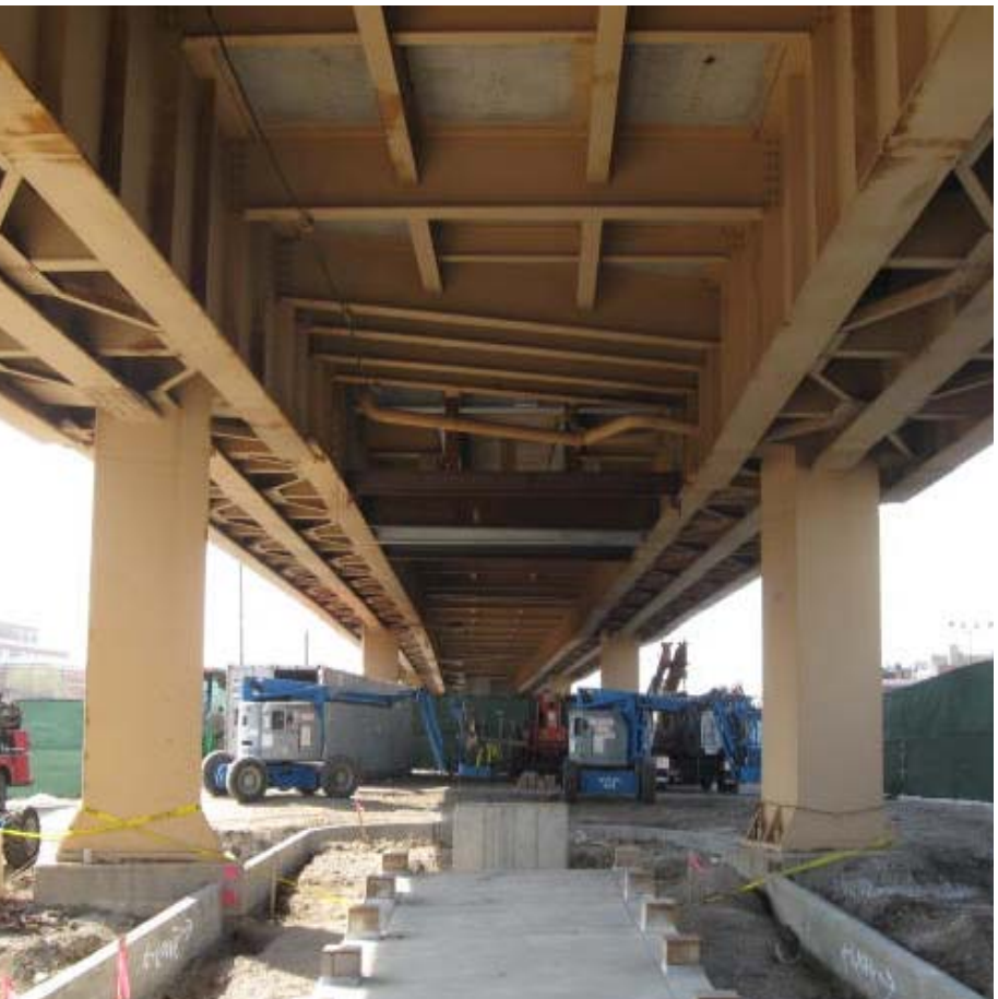
Structural steel in place; framing out new platform staircase to Archer stationhouse.
