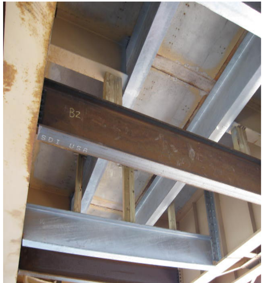
Structural steel in place; framing out new platform staircase to Archer stationhouse.
