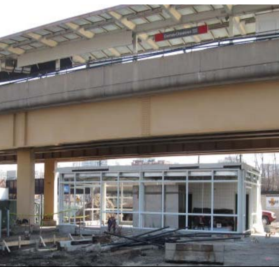
Archer stationhouse steel erected and being built out for passenger use.
