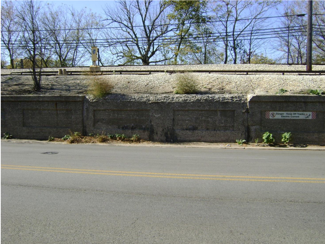
Chicago Avenue wall before construction
