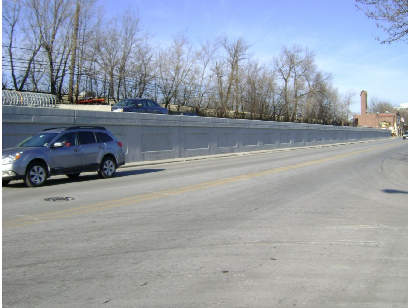
Chicago Avenue Wall Completed
