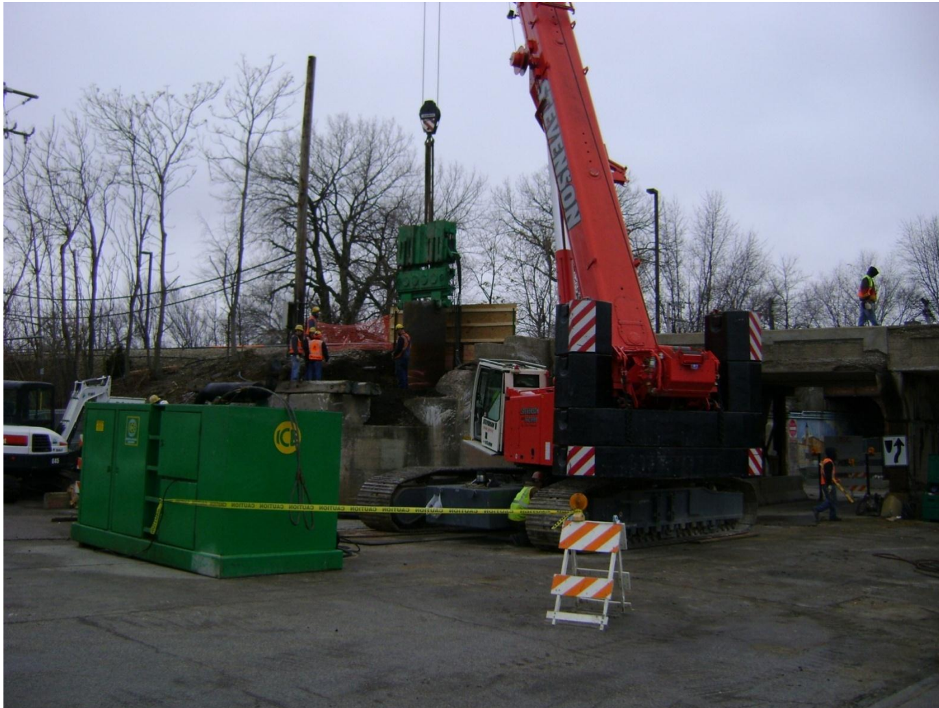
Installing Earth Retention at Greenleaf
