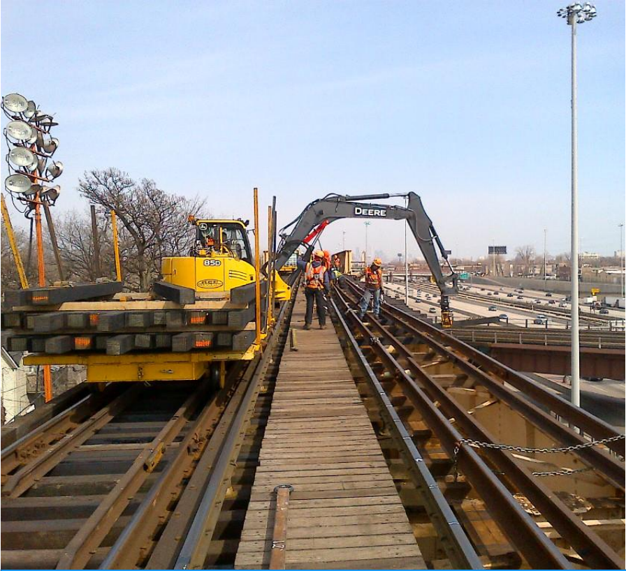
Englewood Track Renewal
