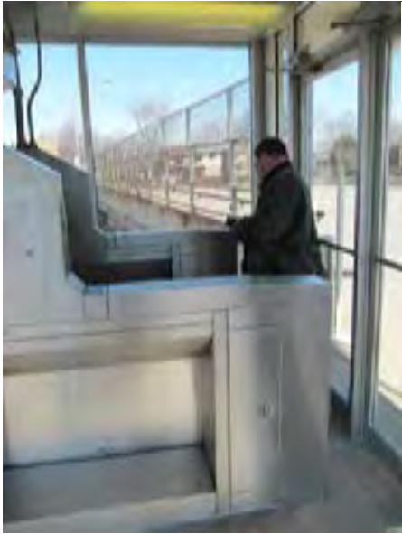
View of secondary station entry at East Avenue, note the narrow distance between the doors and the fare equipment
