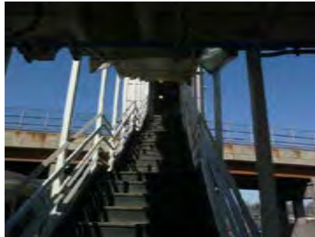
View of secondary station entry stairs at Circle Avenue
