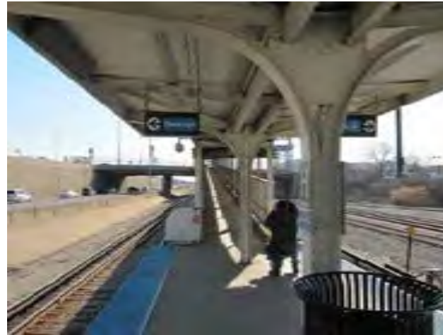
View of exit ramp at east end of platform
