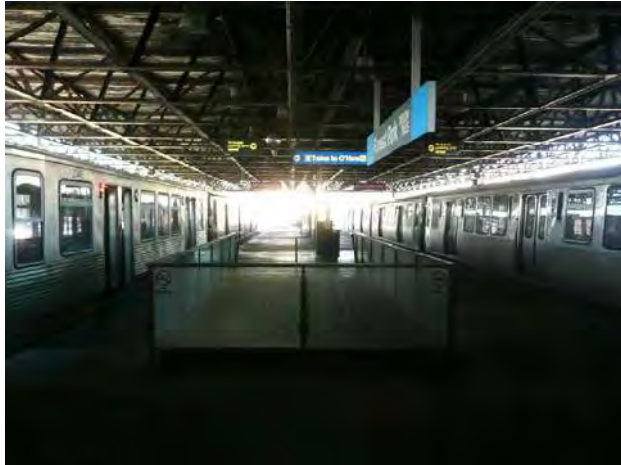
View of exit stair at west portion of platform
