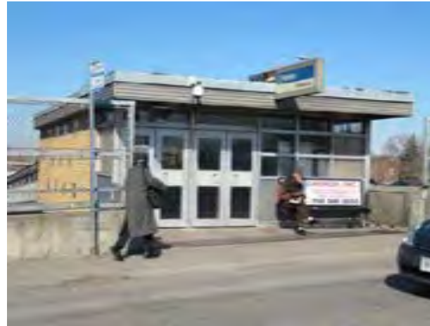
View of main station entry at Harlem Avenue
