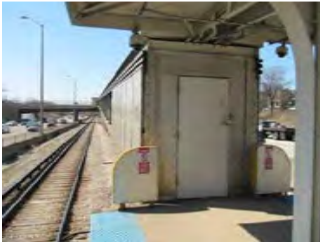
View of closed exit at west end of platform
