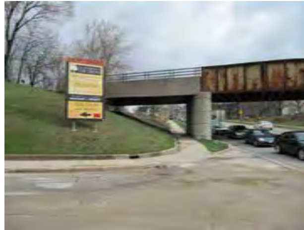
View pedestrian crosswalk area at north side approach to station. Note curb cuts are not ADA compliant and crosswalk is not marked.
