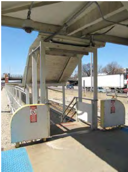
View of exit stair and walkway at west end of platform
