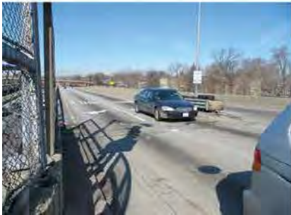
EISENHOWER RAMPS WEST
