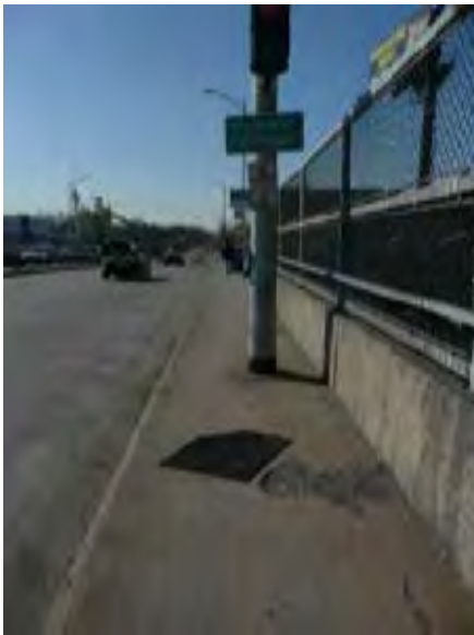
View of signal post impeding sidewalk along Harlem Avenue on approach to station
