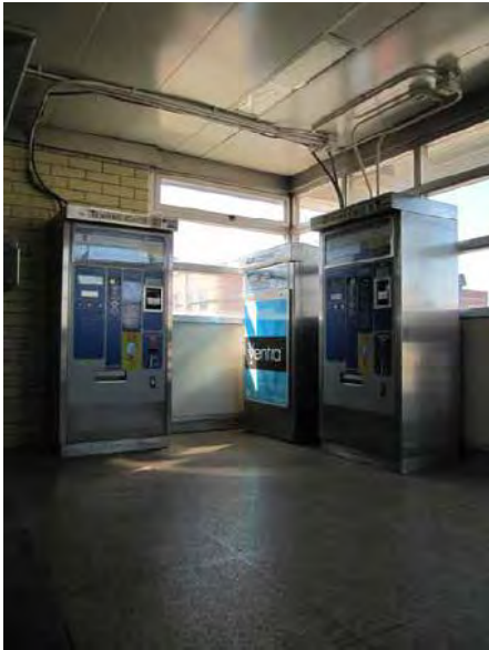
View of main stationhouse interior at Oak Park Avenue
