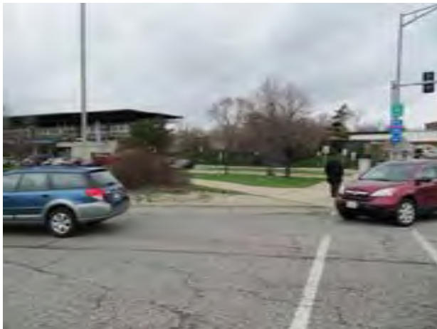
View of crosswalk at south side entry ramp to I-290 on approach to station. Note curb cuts are not ADA compliant, crosswalk markings should be improved and pedestrian signals should be added.
