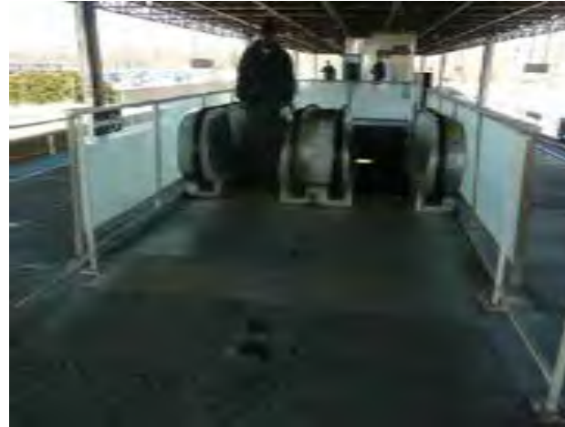
View of escalators at east portion of platform
