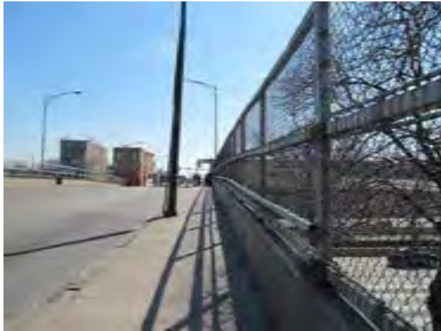
View of sidewalk along Pulaski Road on approach to station
