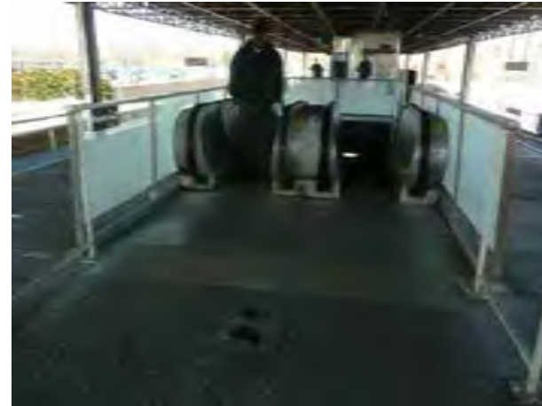
View of escalators at platform level at Forest Park Station
