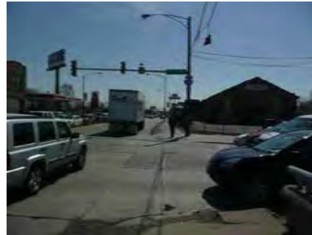
View of crosswalk and curb ramp at Cicero and Lexington intersection. Note broken sidewalk curb ramp that should be repaired.
