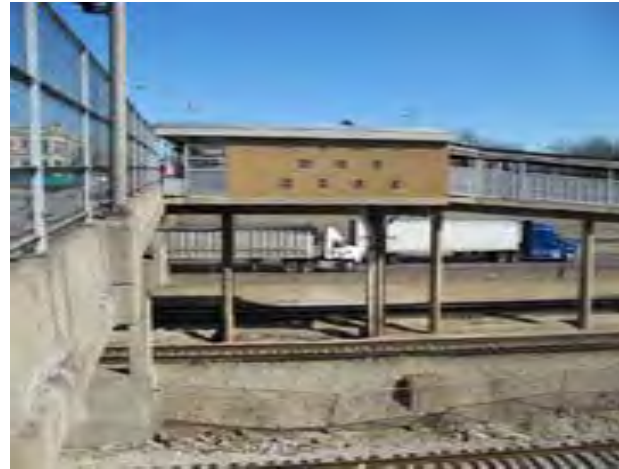
View of main stationhouse entry at Oak Park Avenue
