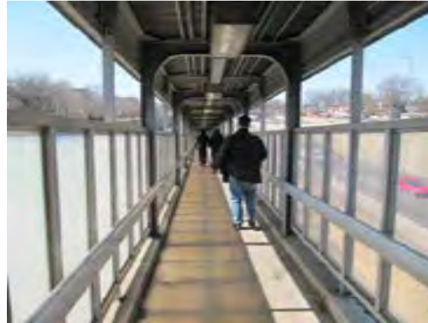
View of main station entry ramp at Austin Avenue
