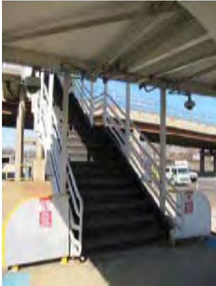
View of exit stair at west end of platform
