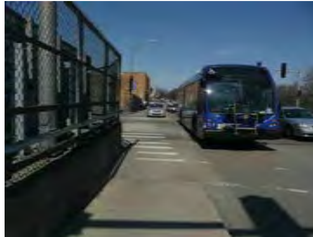
View of non-compliant curb ramp at Austin Avenue on approach to station.
