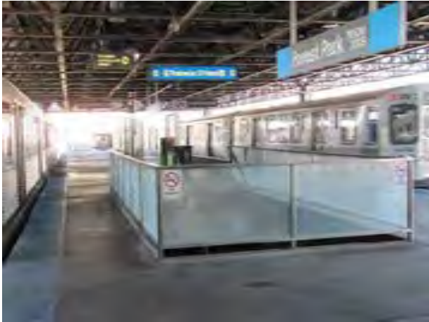
View of stair enclosure at platform level at Forest Park Station
