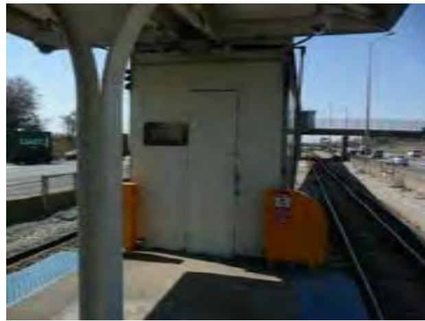
View of secondary station entry ramped closed at Lavergne Avenue pedestrian bridge
