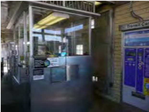
View of main stationhouse interior at Oak Park Avenue
