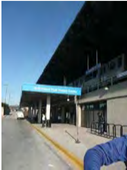
View of main station south entry at Forest Park Transit Center
