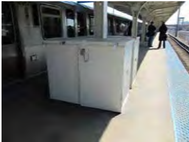
View of non-compliant platform with impeding elements
