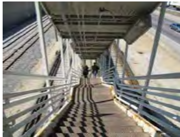
View of secondary station entry stairs at East Avenue
