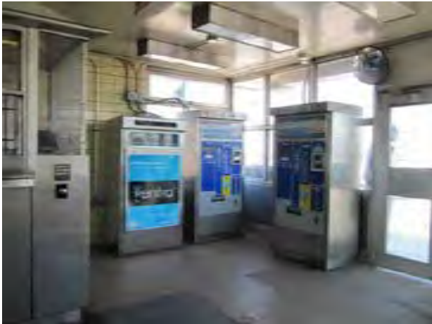
View of main station interior at Pulaski Road
