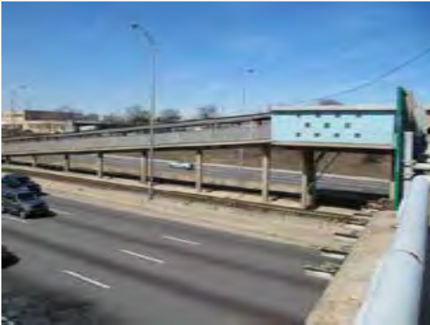
View of main station house and entry ramp at Cicero Avenue
