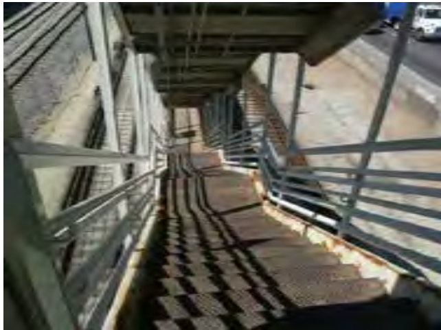
View of exit stair at east end of platform
