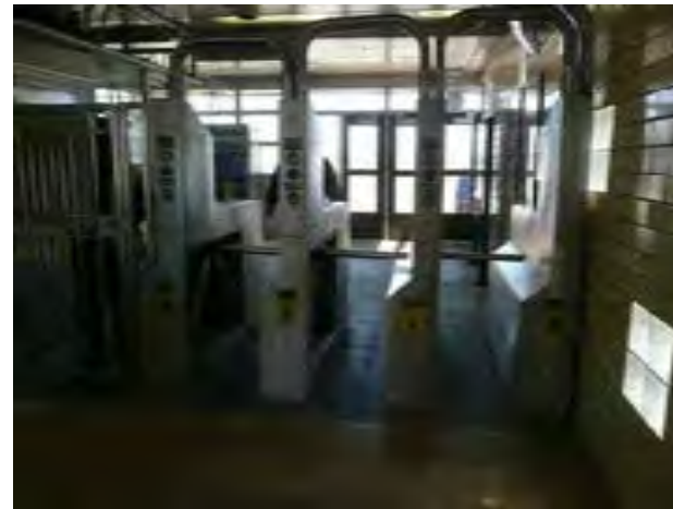
View of non-compliant fare array and entry doors beyond at Austin Avenue Station
