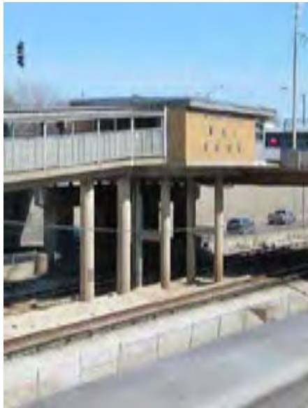
View of main stationhouse building at Austin Avenue
