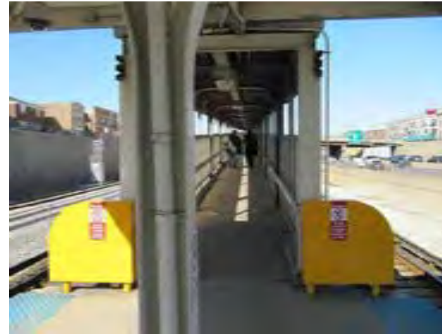
View of exit ramp at west end of platform
