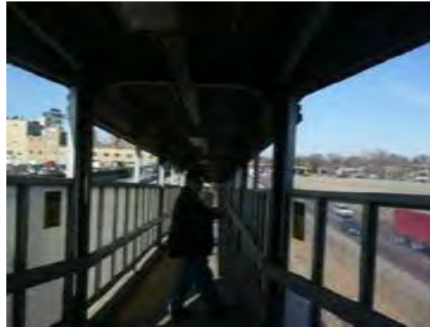
View of main station entry ramp at Harlem Avenue
