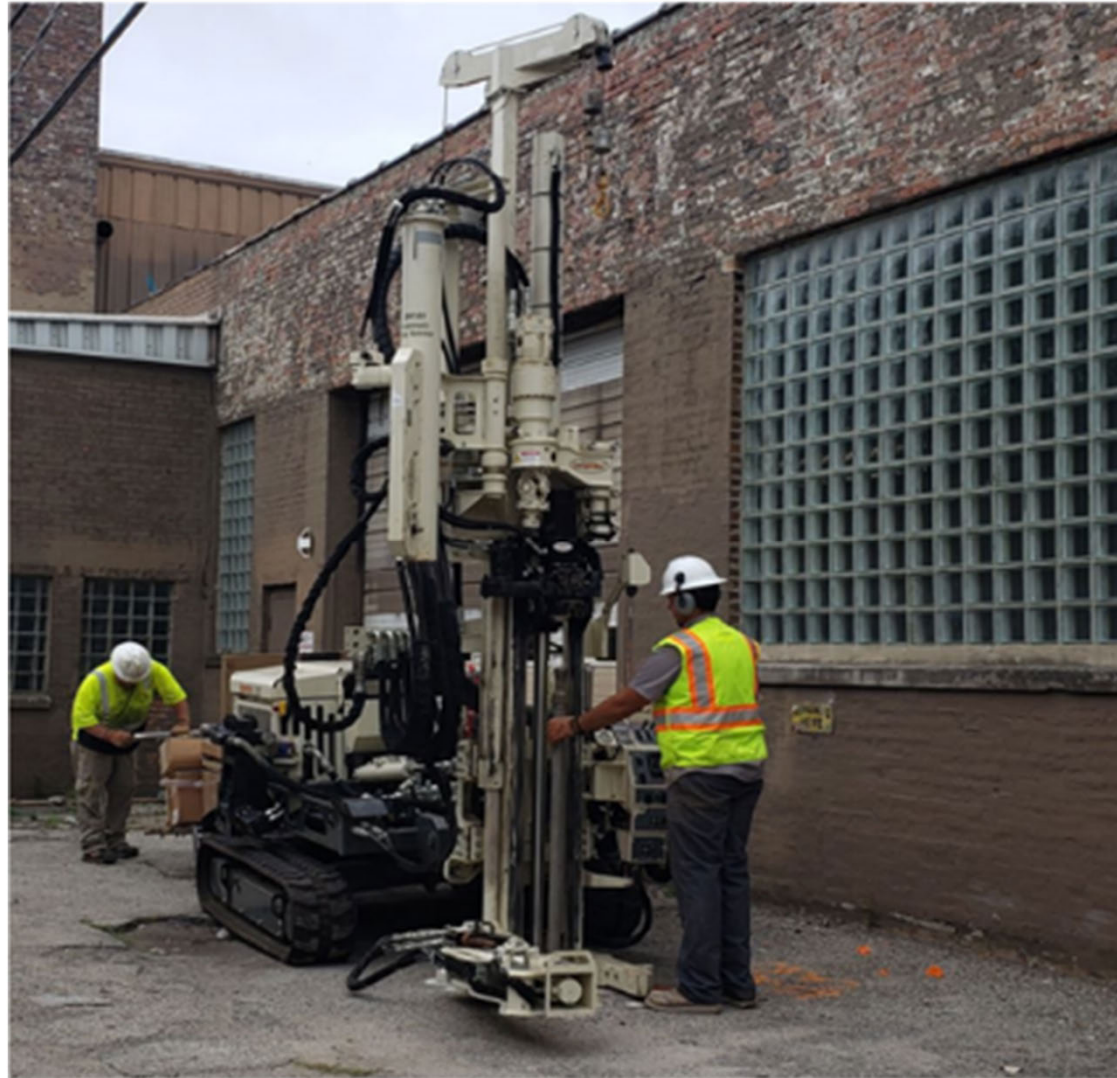
Lawrence to Bryn Mawr Modernization – Geotechnical soil borings
