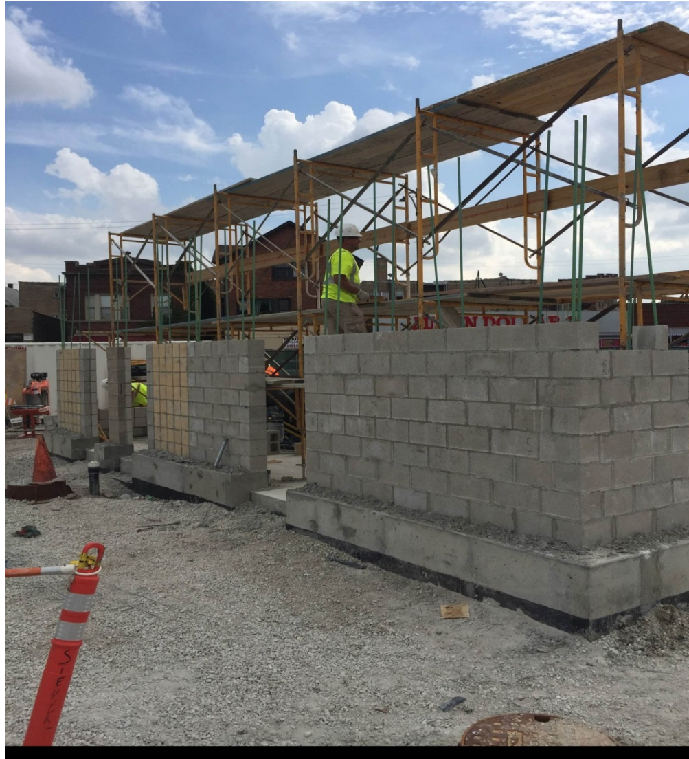
Chicago/Austin – Masonry Installation
