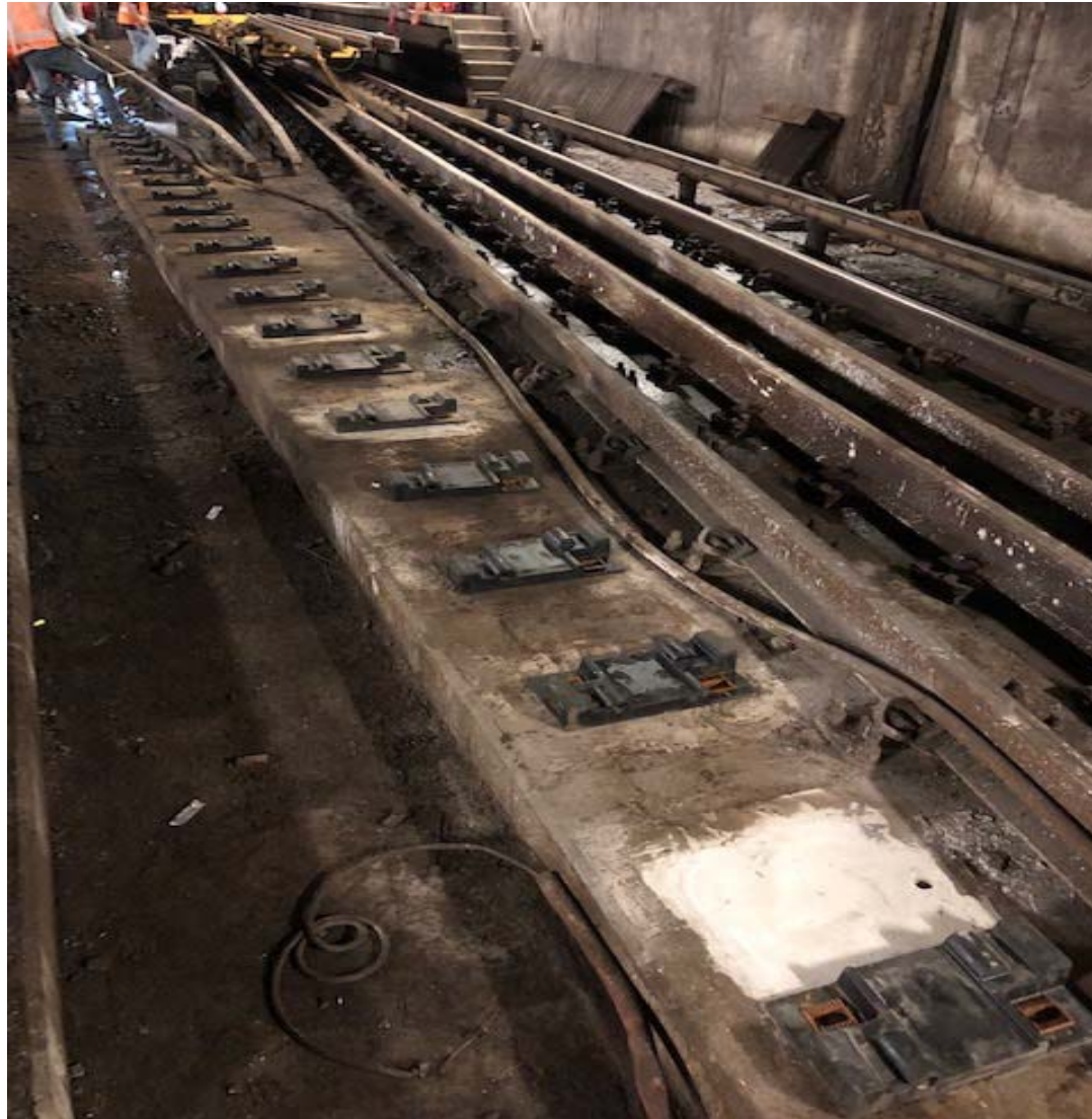
Track Plate Installation
