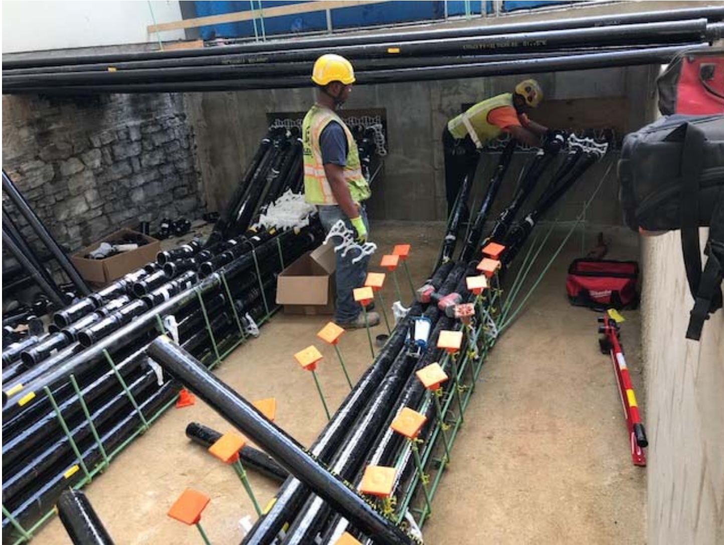
Exterior Ductbank Installation at East Lake Substation
