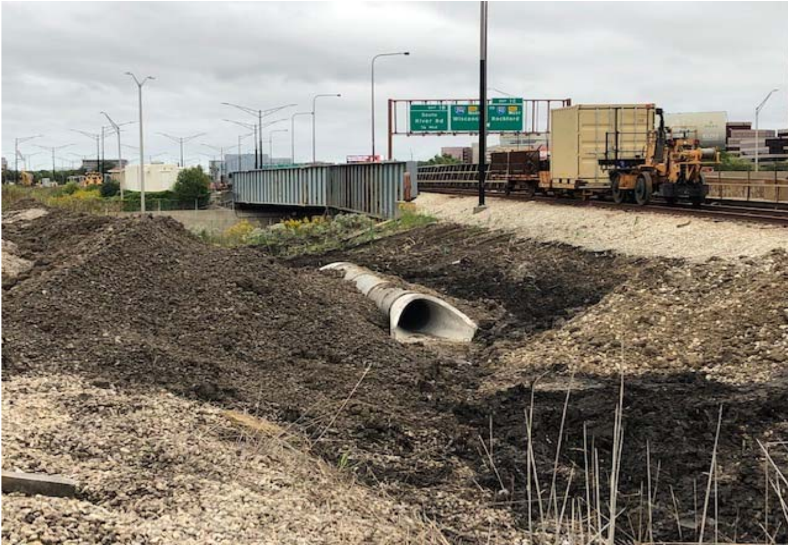
Grading for future Relay House installation
