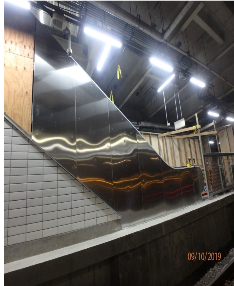
Installing SS Cladding on east Side of escalator 1
