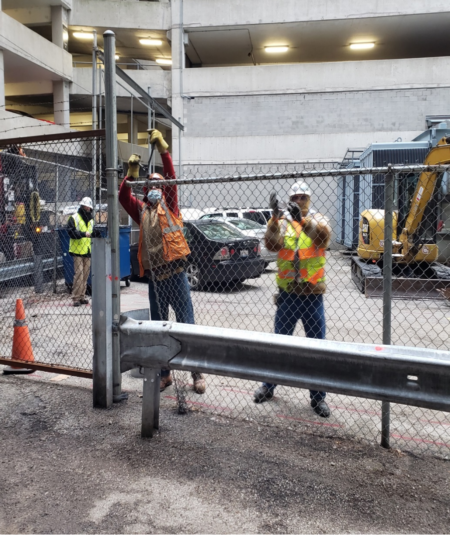
Removing Existing Fence at Franklin Substation
