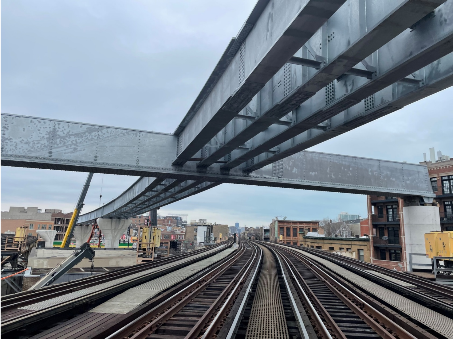
RPB - Straddle Beam and Girders Installation
