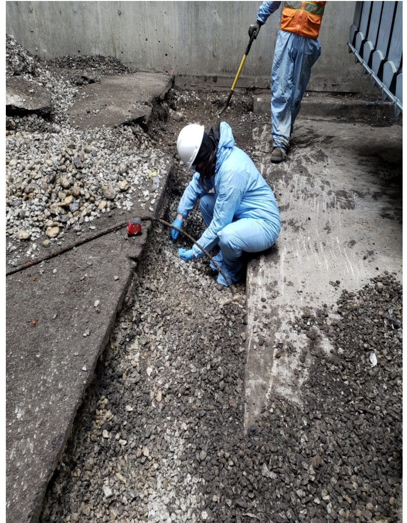
Taking Soil Samples at Franklin Substation
