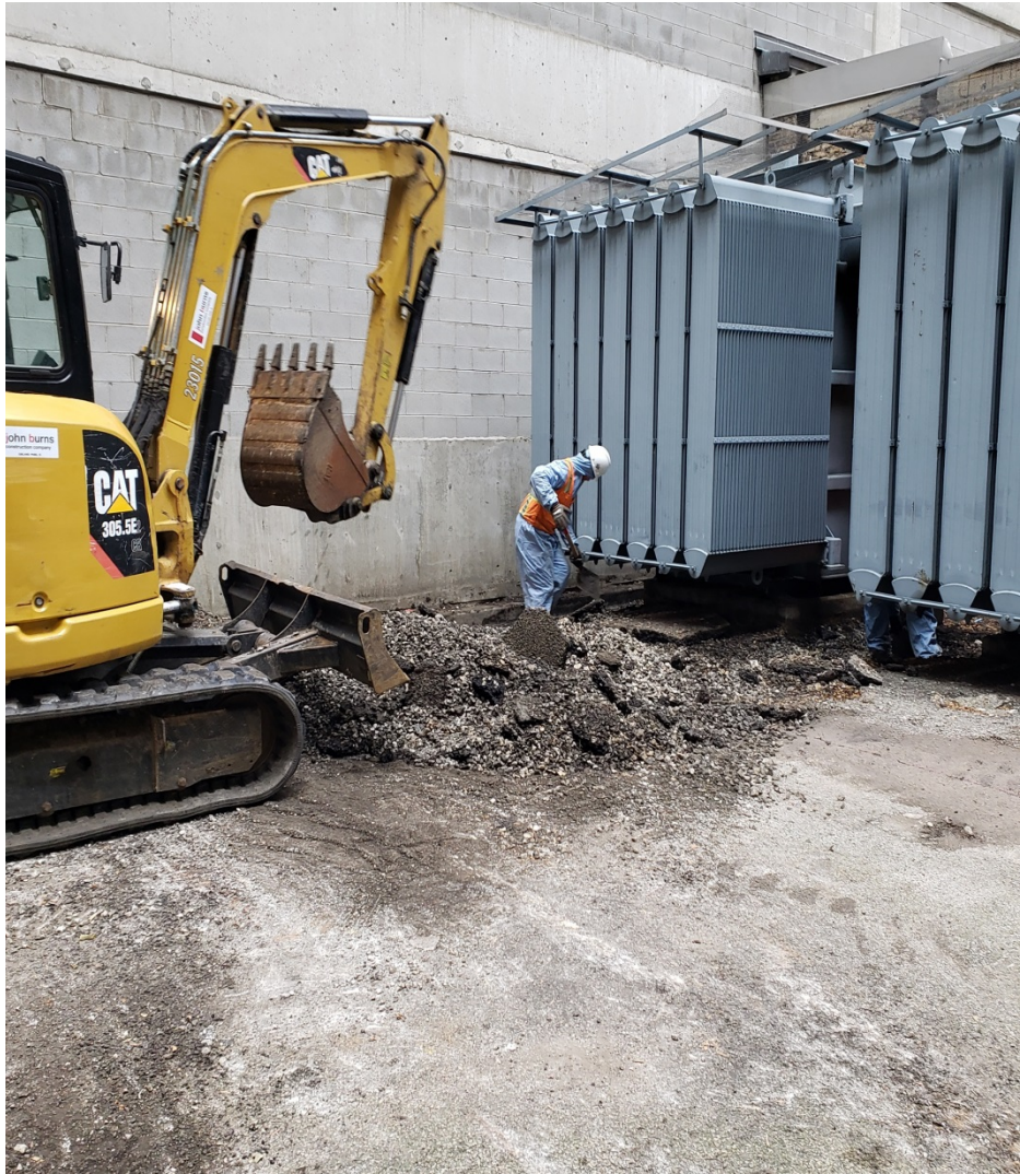
Excavating Around TX1 at Franklin Substation
