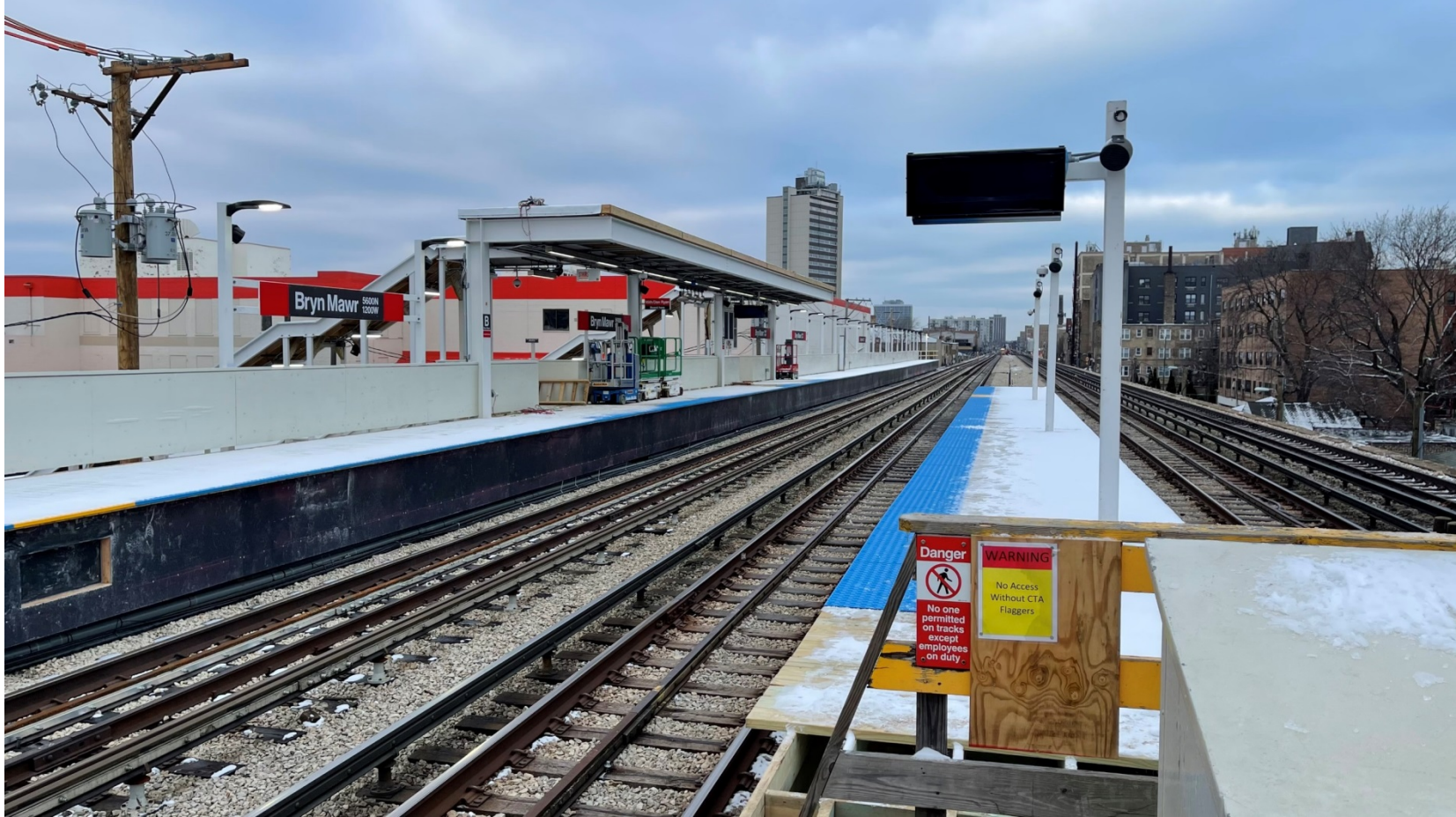
LBMM - Bryn Mawr Temporary Station Platform
