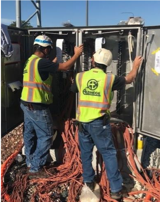
Cable Termination in Rosemont Yard and Rosemont Relay Room
