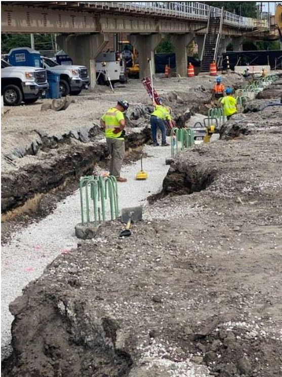
Flood Performing Density Compaction Testing
