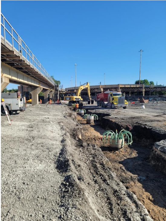
Grade Beam and Pile Cap Excavation
