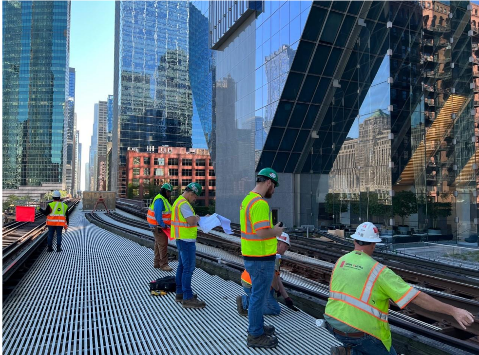
Canal Tie House Site Layout Field Verification
