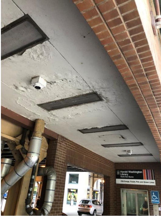
Harold Washington/Library- Repair water damaged ceiling and repaint
