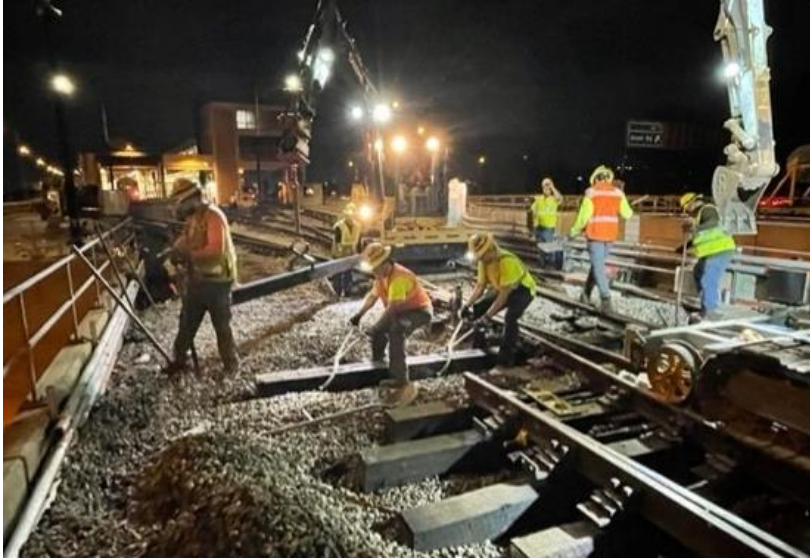
Special Trackwork Installation at Rosemont Yard
