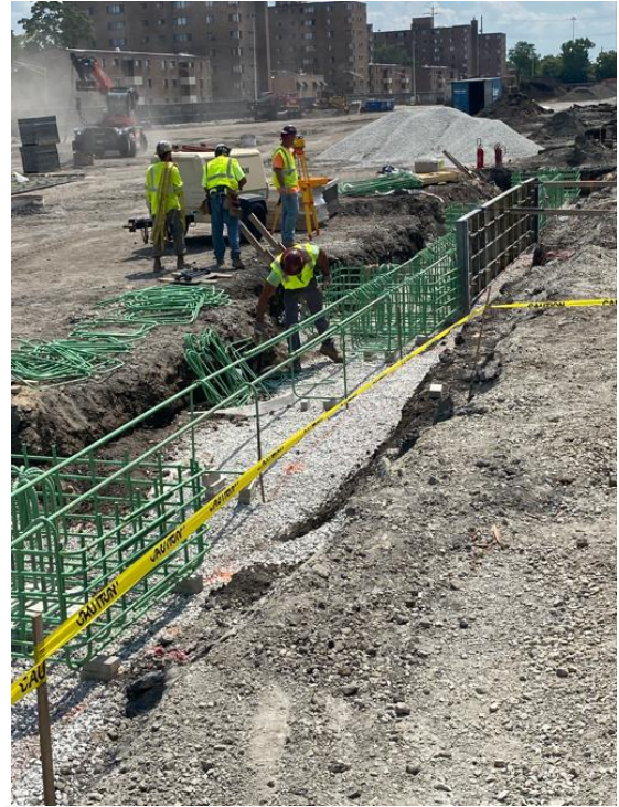
Grade Beam and Pile Cap Excavation
