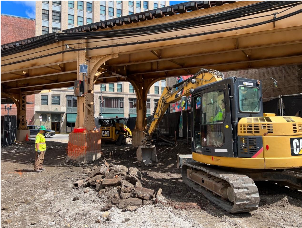
Old Foundation Removal At Damen
