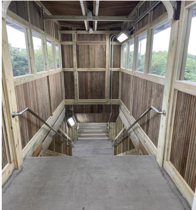
Beadboard Panel Install
