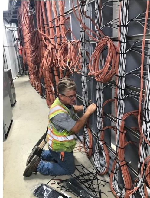
Cable Termination in Rosemont Yard and Rosemont Relay Room
