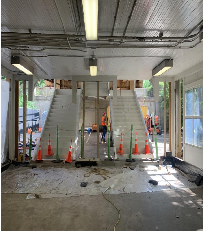
Lower Stairwell Installation
