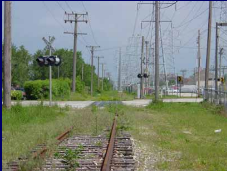
Gross Point Rd. looking North
