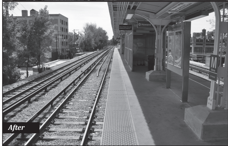
Seven Red Line stations on the North Side received much-needed capital maintenance and upgrades as part of the North Red Interim Station Improvement Project, including the Morse Red Line station, which reopened in August 2012 with new concrete platforms, refurbished canopies and new fixtures and signage.
