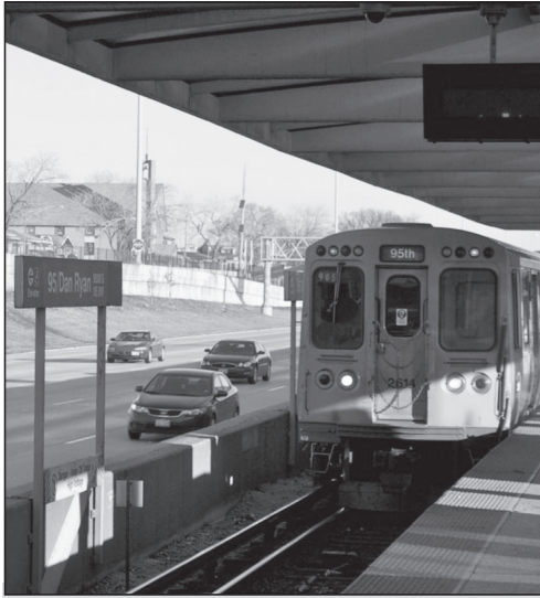
Reconstruction of Red Line South between 22nd and 95th Street will begin in May 2013 and will dramatically improve aging stations and infrastructure for a quicker, more comfortable commute.
