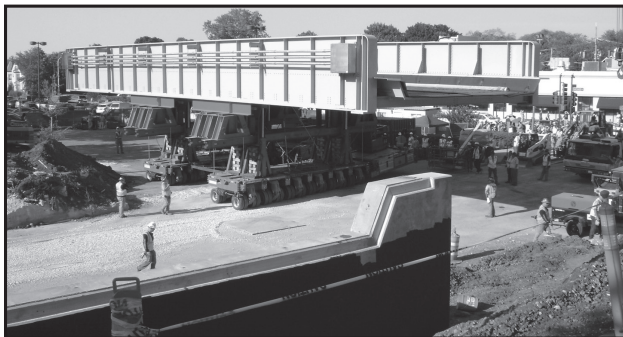
The CTA is committed to dramatically reducing the number of slow zones across its system. In 2012 CTA replaced three viaducts on the Purple Line that were more than 100 years old that were contributing to longer travel times for customers.
