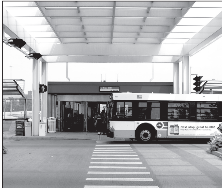
During the reconstruction of the Red Line South, CTA will provide free bus shuttle service to help customers get to their destinations and provide significant additional bus service on routes within the project area.
