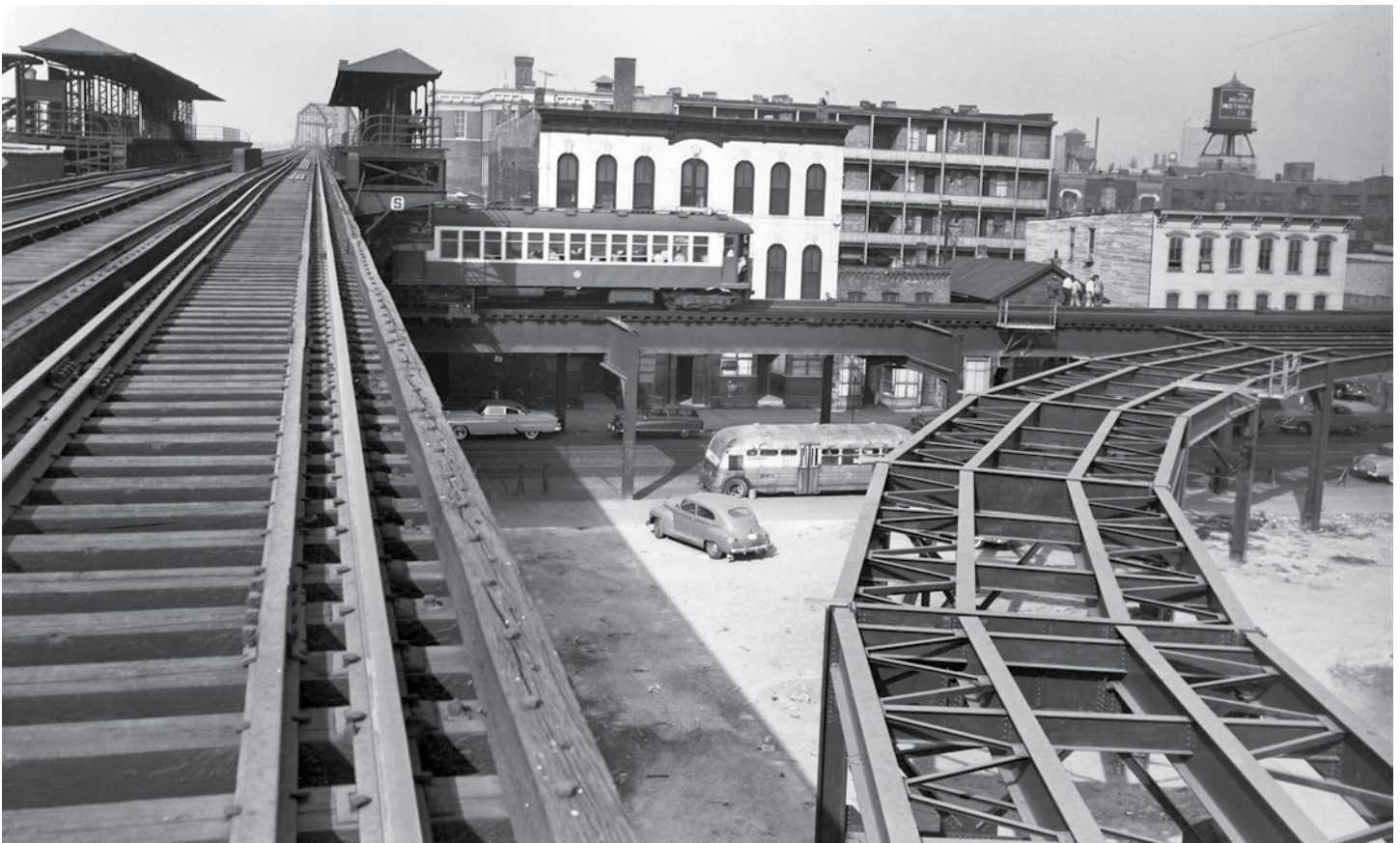
A Loop-bound Lake Street train consisting of 4000-series cars, led by a "Plushie" type car (built by the Cincinnati Car Company between 1922 and 1924), travels east. Pictured above it are the original Logan Square 'L' tracks and the Lake Street Transfer station, no longer in use at the time of the photo. Under construction is the connection between the two routes to form what would eventually become known as the Paulina Connector. The Connector allowed Douglas Park trains to reach the Loop during the 1954-58 period when its old route to the Loop was demolished to allow for construction of the Eisenhower Expressway and the Congress rapid transit line. Today, the connector is used by Pink Line trains to and from the Loop.
