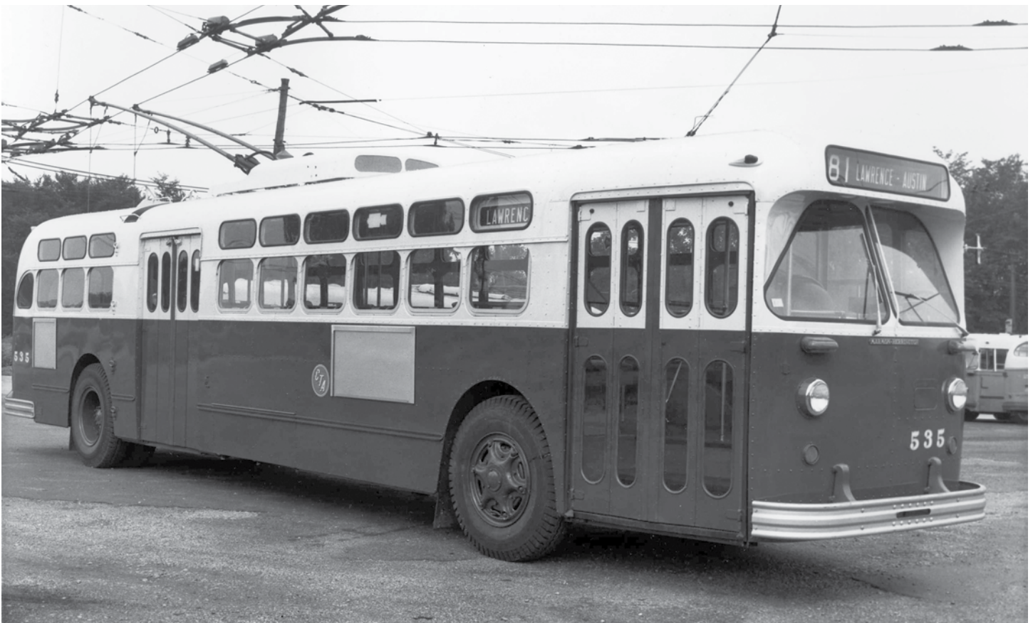
CTA trolley bus #535 (built by the Marmon-Harrington Company in 1951 and later renumbered #9535) had just recently been delivered and was assigned to the #81 Lawrence route. Three-hundred and forty-nine trolley buses of this type were delivered between 1951 and 1952, and operated on various routes until the end of trolley bus service in March of 1973. A number of these buses were sold to Guadalajara, Mexico, where they remained in service until 1993.
