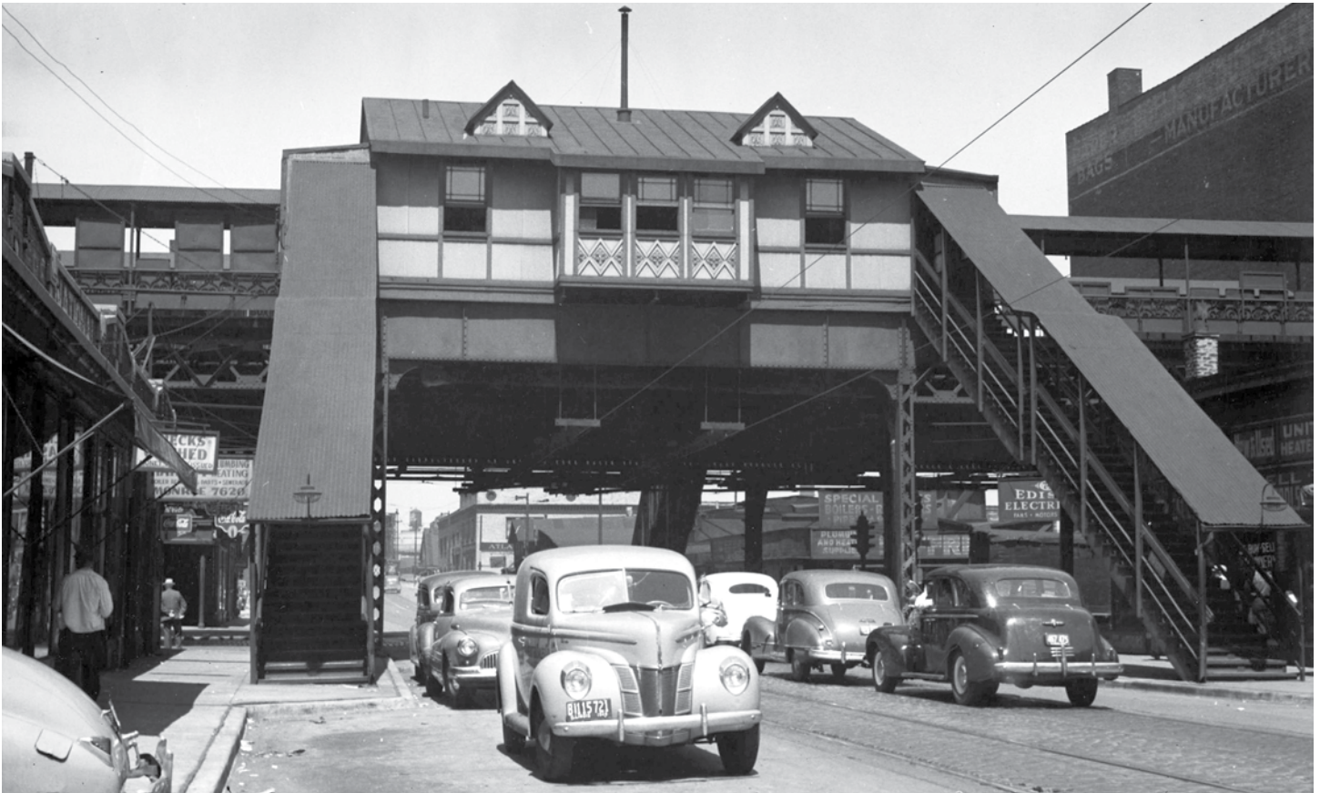
A mid-1940s view of the Lake Street Elevated Halsted station looking north on Halsted at Lake. The station was demolished in 1994 during the Green Line renovation. Similar stations remain in service today on the Green Line at Ashland/Lake and Conservatory-Central Park Drive.
