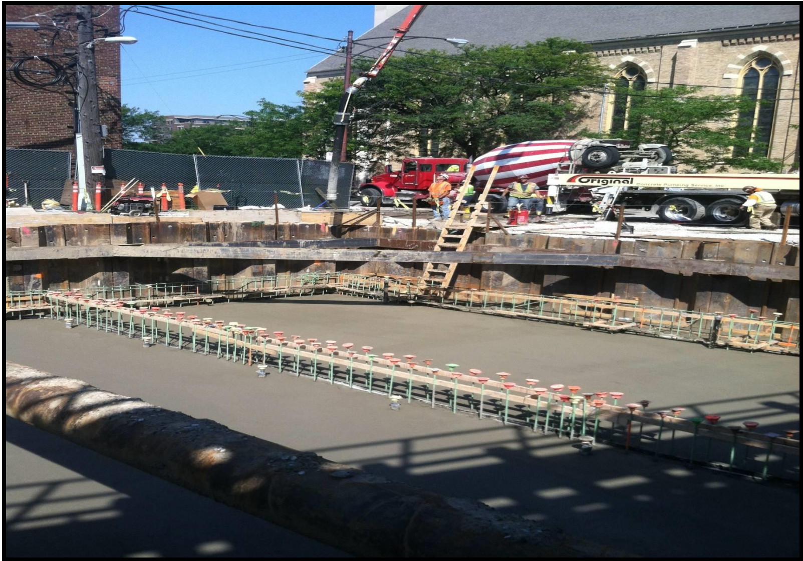
Hill Substation Slab
