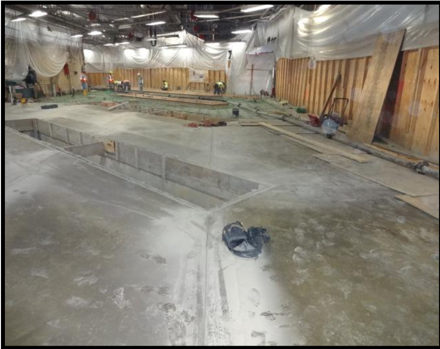
North Park - Paving
