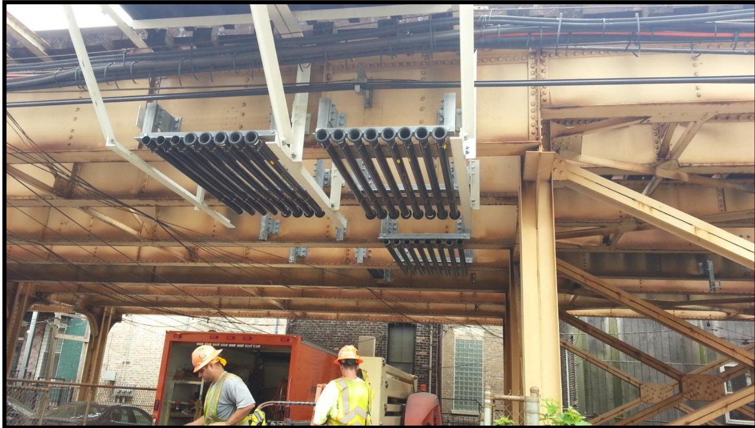
Armitage – Bracket Installation
