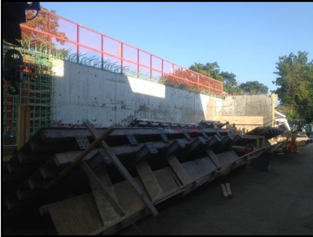
West Wall installed at Farwell Substation
