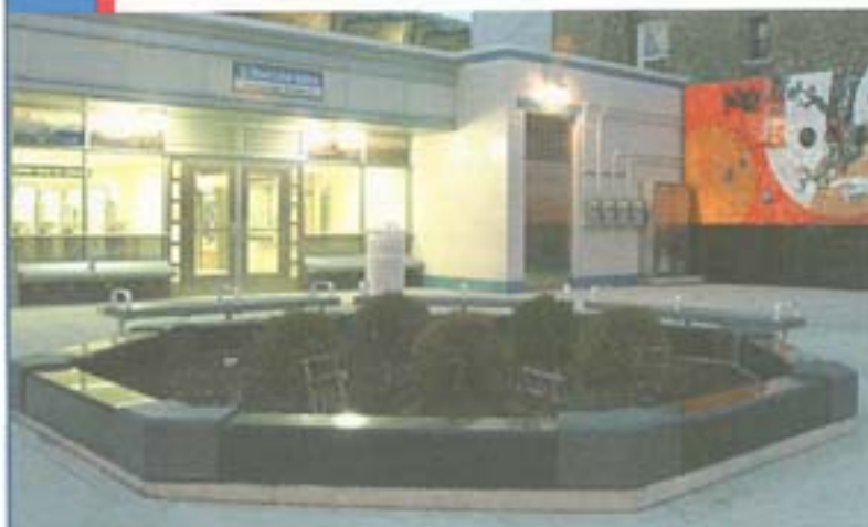
Improved lighting at the Blue Line's newly renovated Damen station on the 54th/Cermak branch lights up the neighborhood at dusk.
