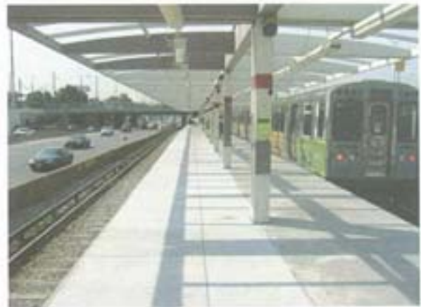
A new concrete platform is one of the upgrades at the Garfield station on the Red Line as part of the rehabilitation of the Dan Ryan branch.
