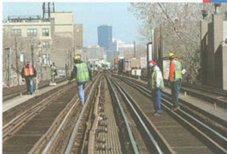
A CTA maintenance crew tends to the elevated tracks near Fullerton.
