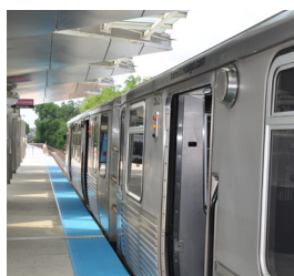
Tactile platform edging
