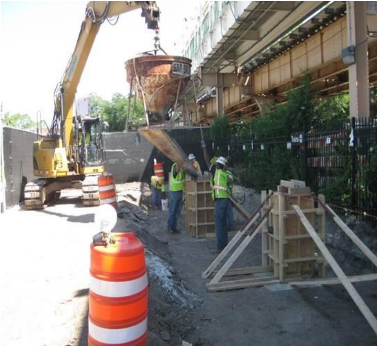
Pouring Concrete in Stair Column Pedestals
