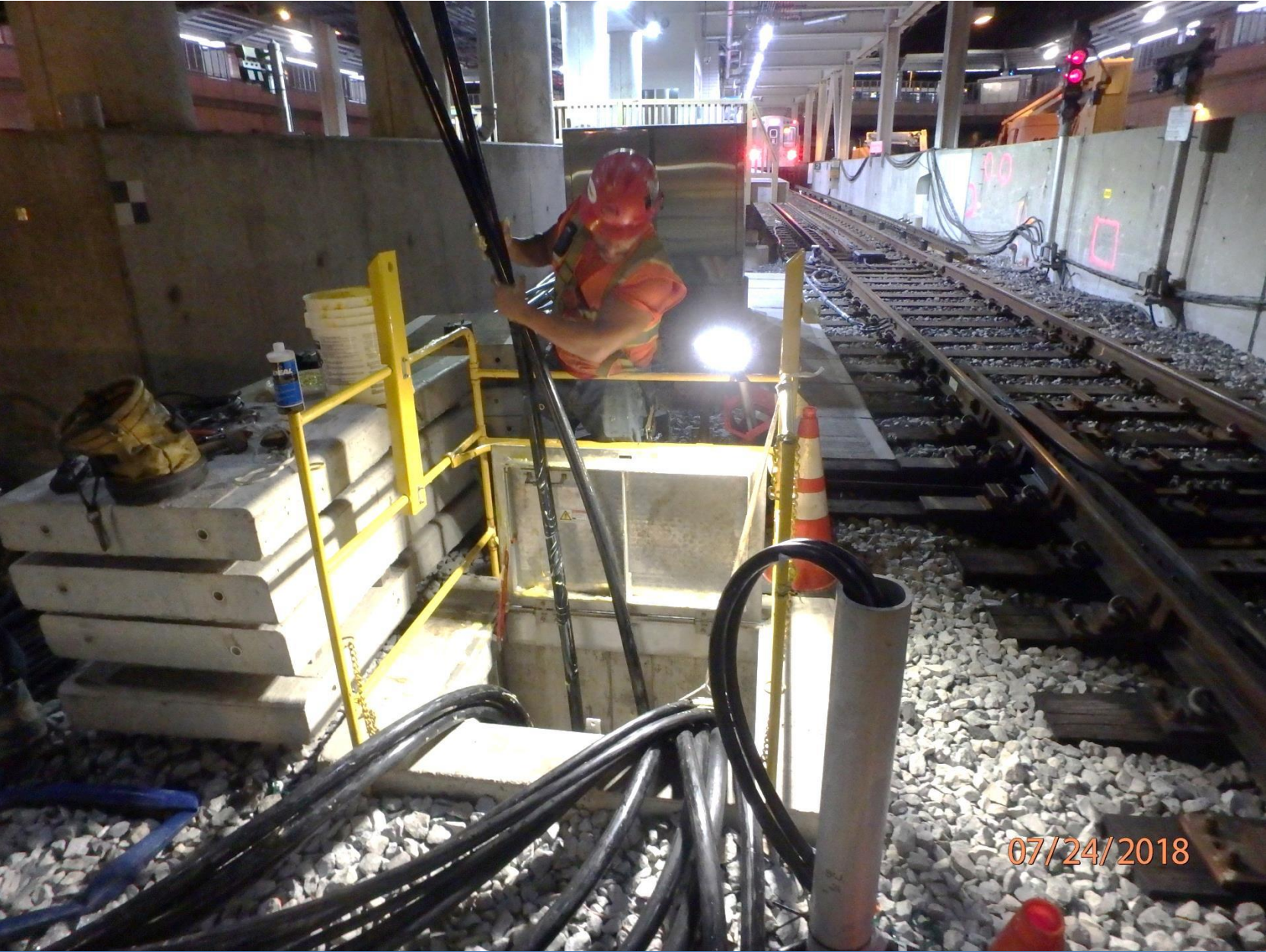
Cable Pull - 96 th Interlocking Signaling System
