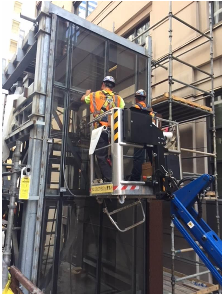
New Elevator Glazing Installation
