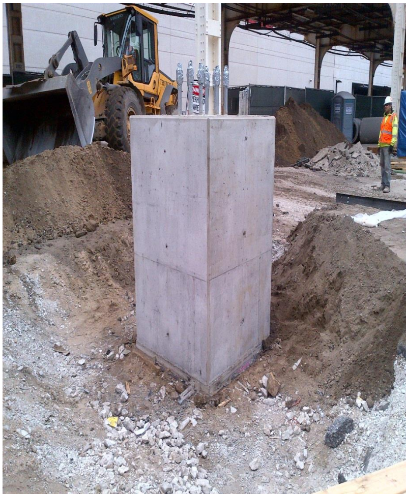
Column Pedestal Installation
