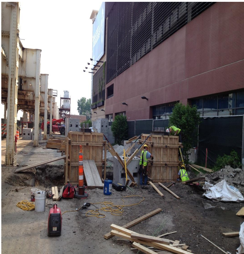
Column Pedestal Installation
