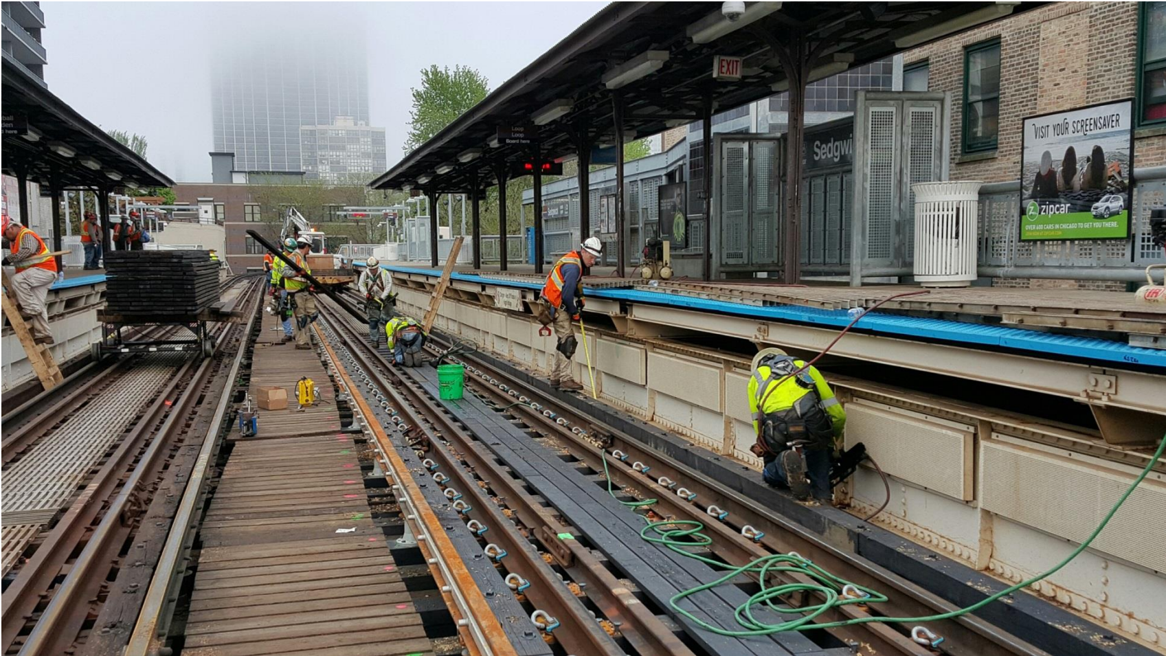
Contractor Placing Track at Sedgwick Station
