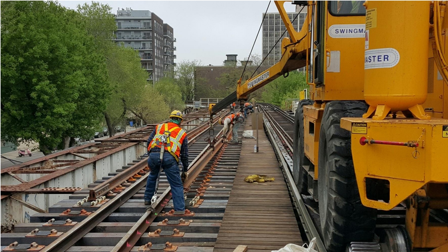
Contractor Installing New Running Rail
