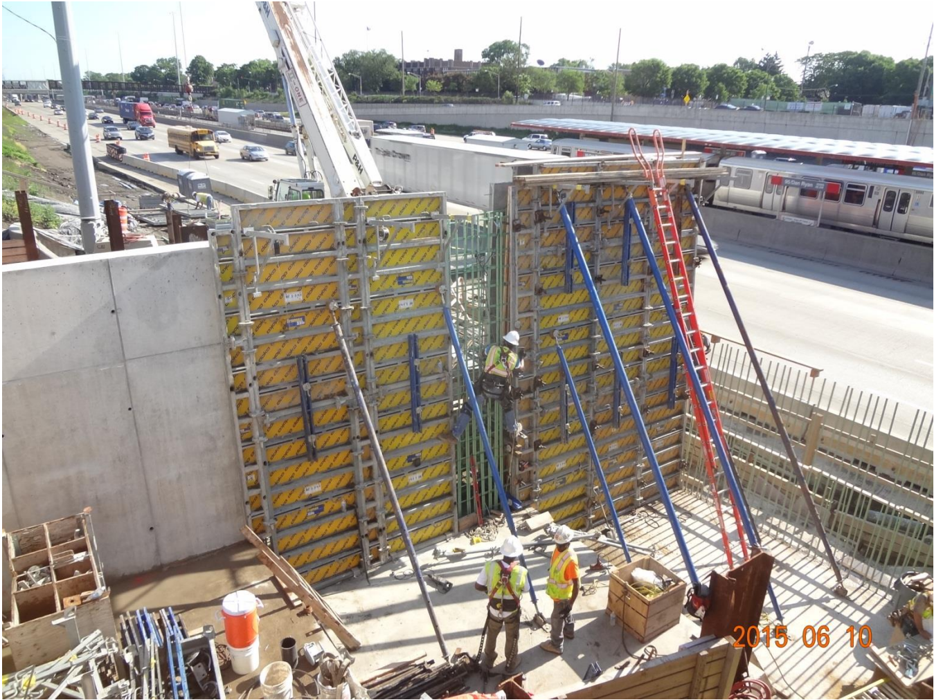
AP2: Form Work at Northwest Quadrant (Wall 2)
