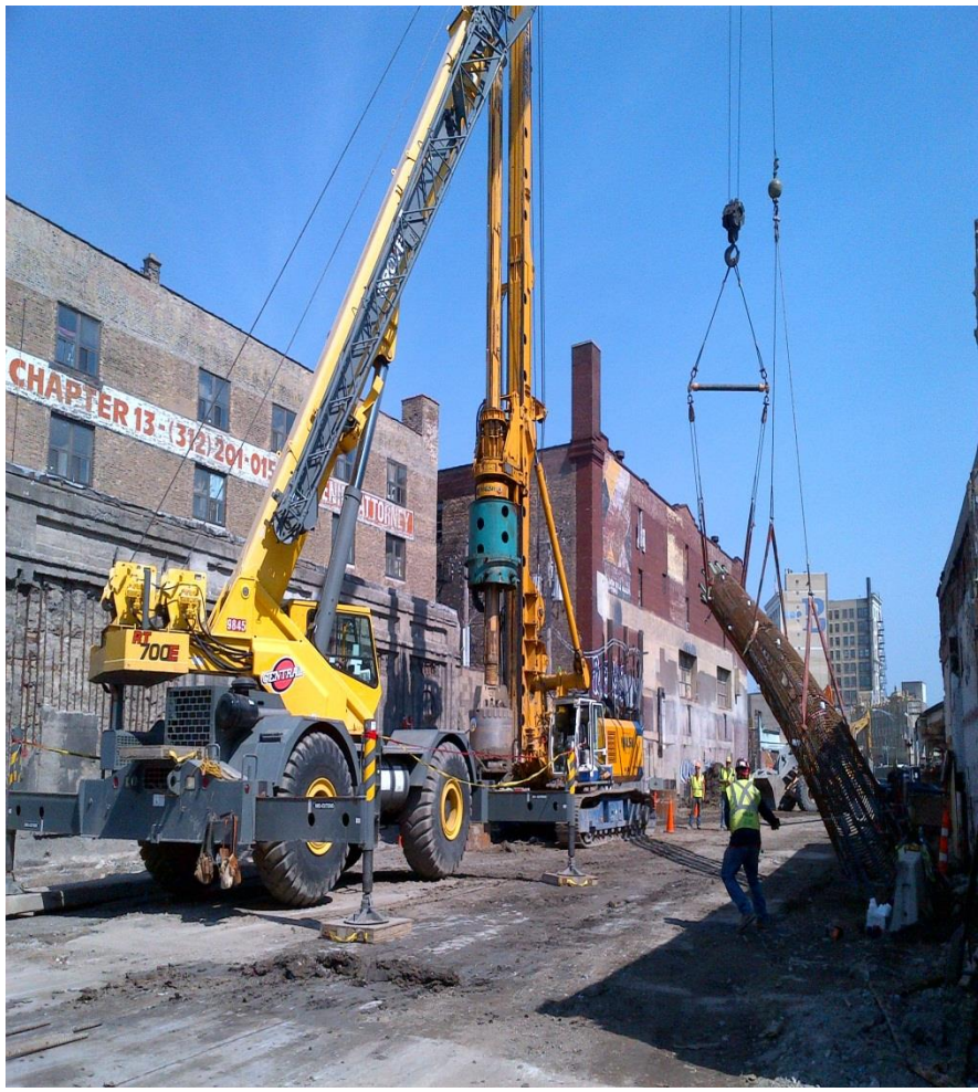
Caisson installation – North of Wilson
