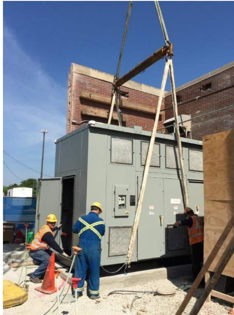
Kimball Substation: Installation of Transformer
