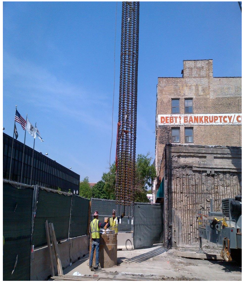
Caisson installation – North of Wilson
