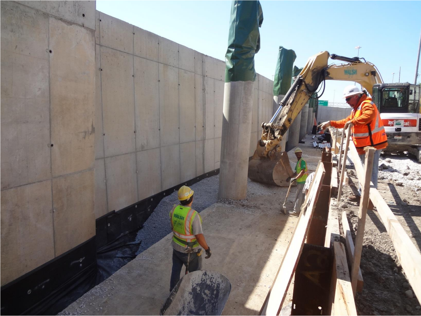
AP2: Backfill Work on Southwest Quadrant (Wall 1)
