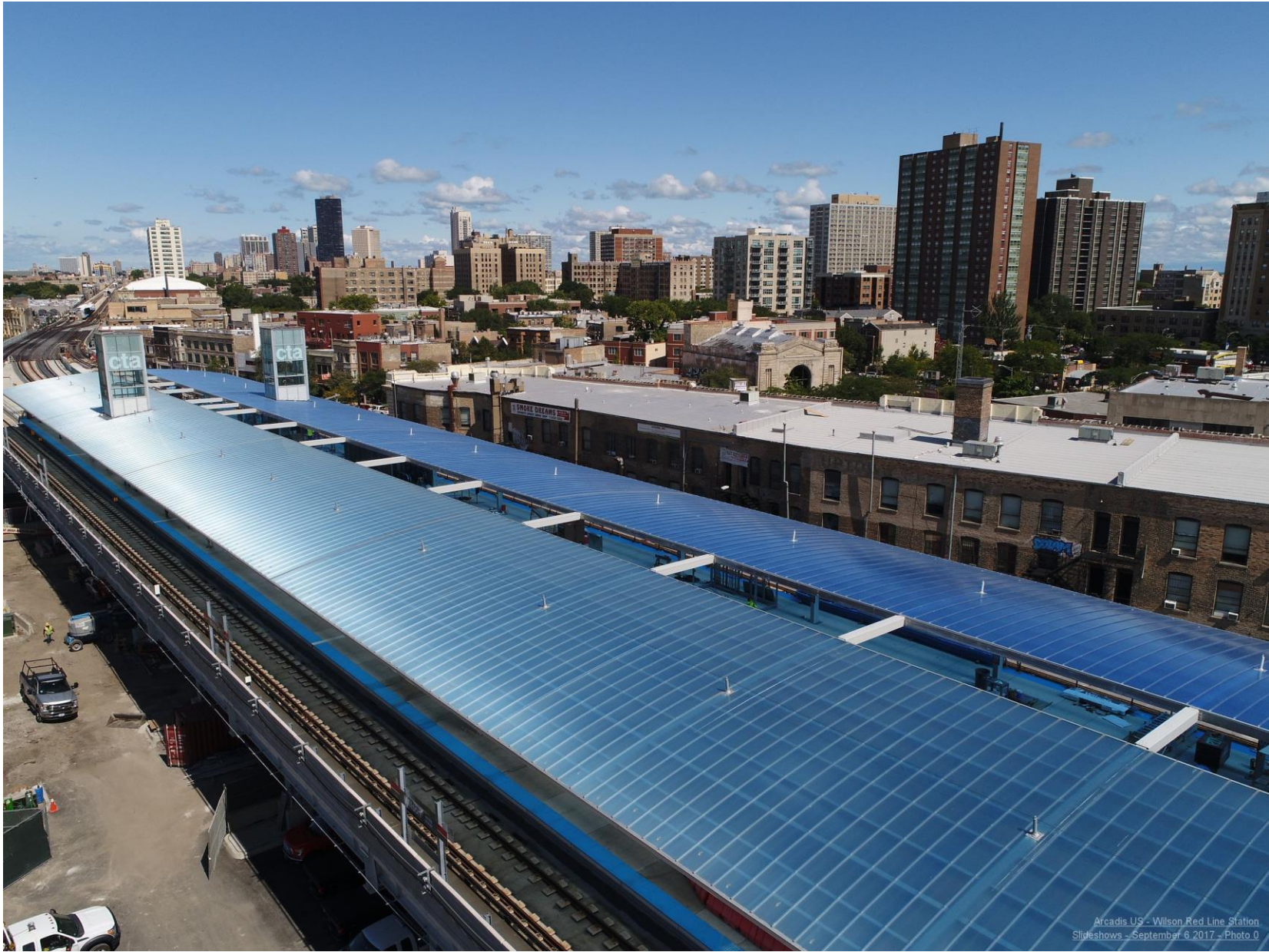
Elevators Towers and Canopy Build Out
