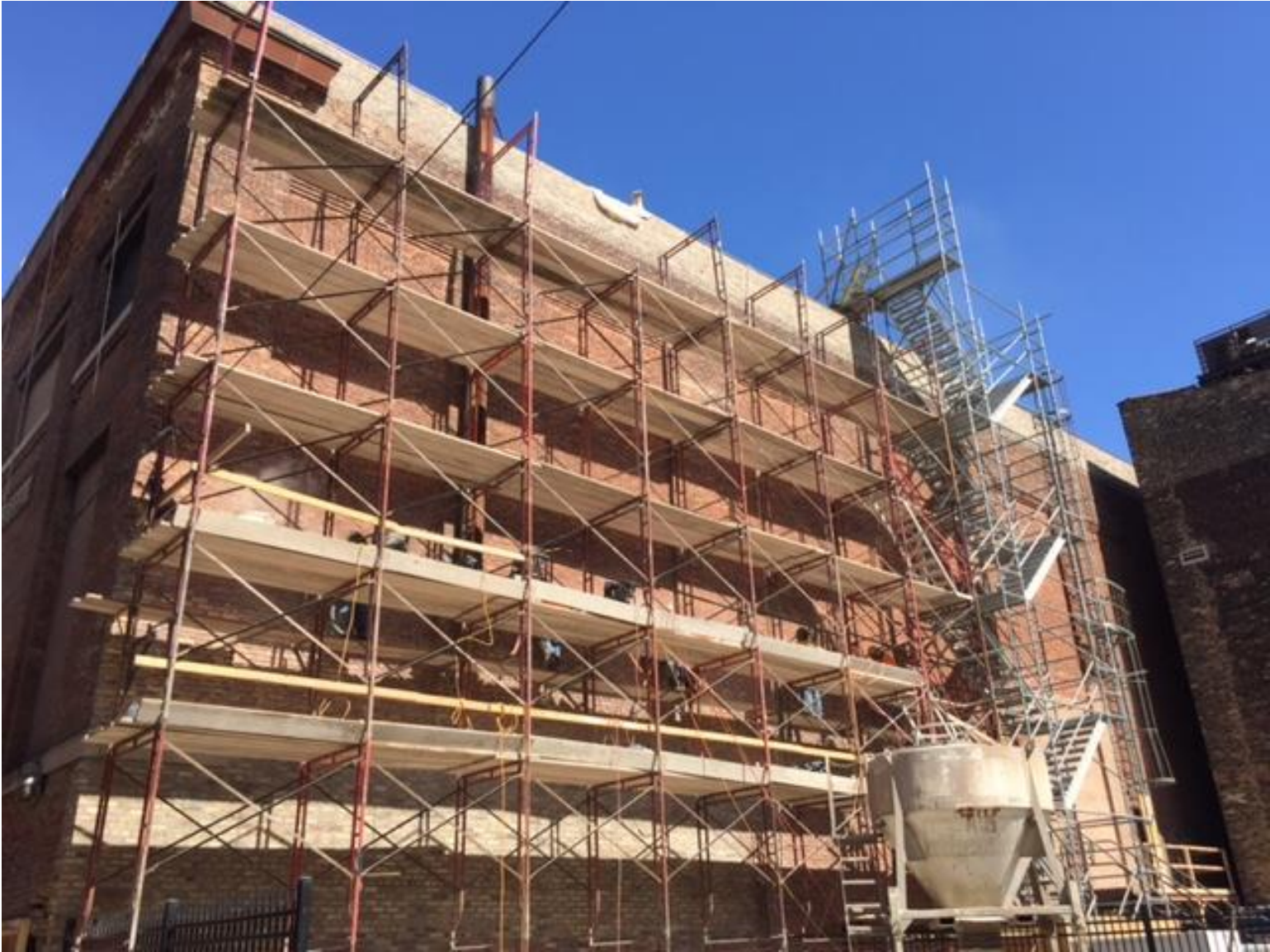
Illinois Substation Tuck-pointing
