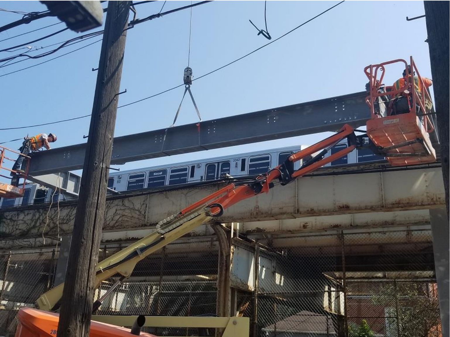
Installing Willow Relay House Platform Steel
