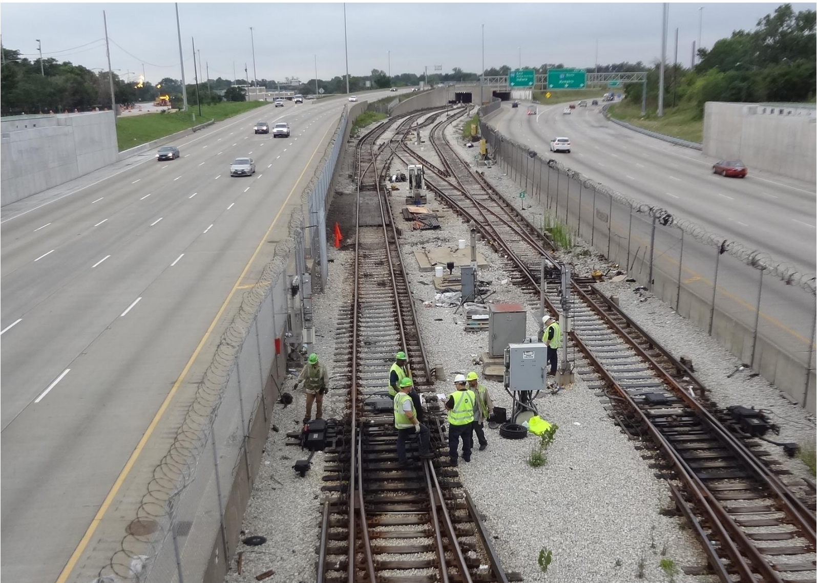
Temporary grade crossing installation
