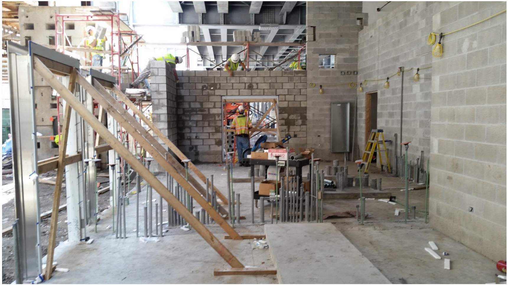
New Wilson station masonry wall installation
