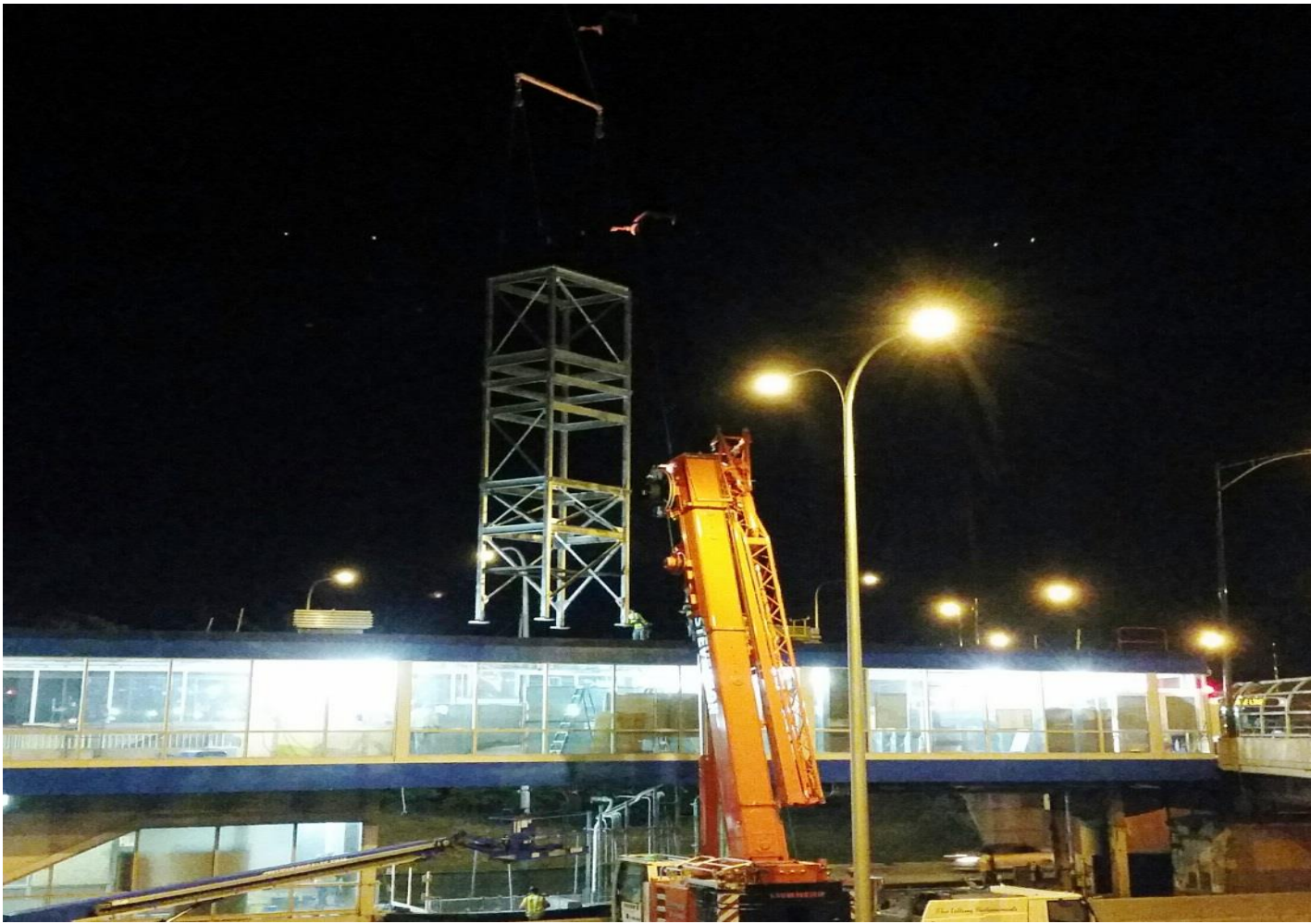
New elevator tower hoisted into Addison Station
