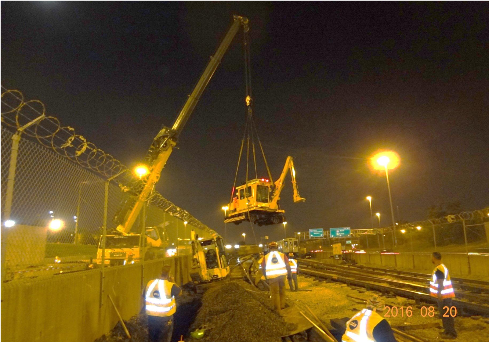
Temporary traction power work
