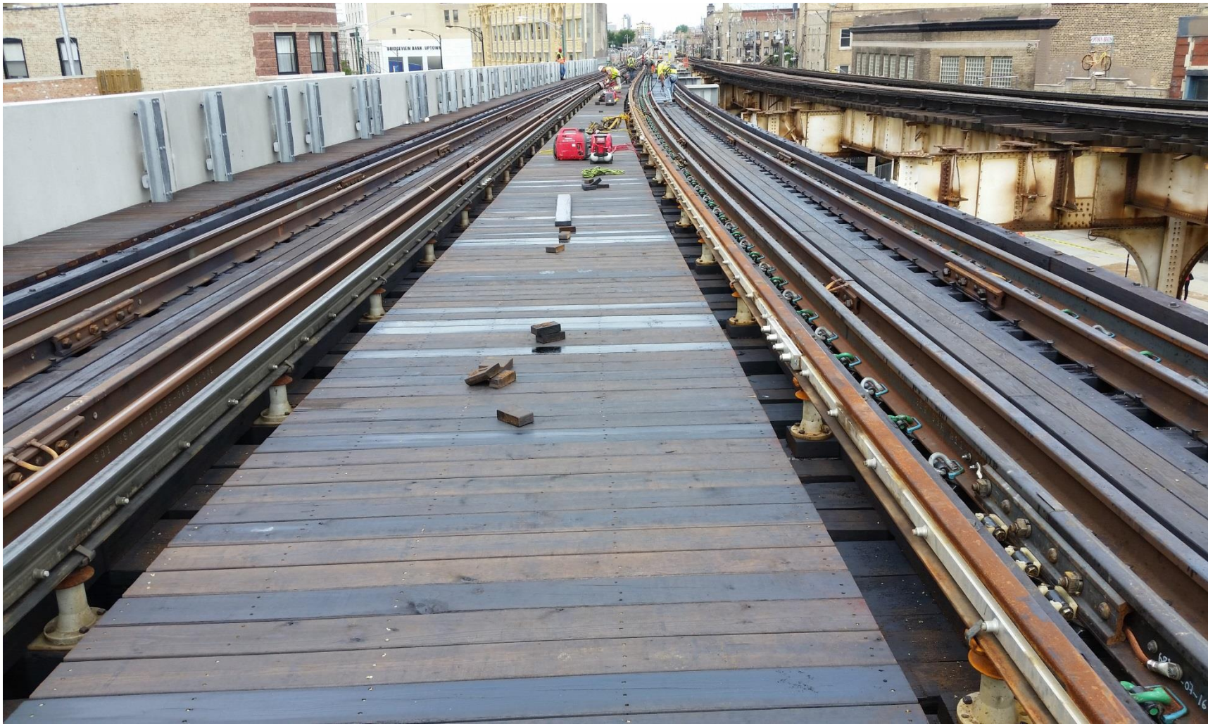
New north section of open deck track 2 and footwalk installation
