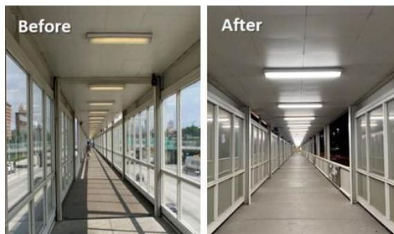
Lighting upgrade in the pedway at the Sox-35 th Red Line Station
