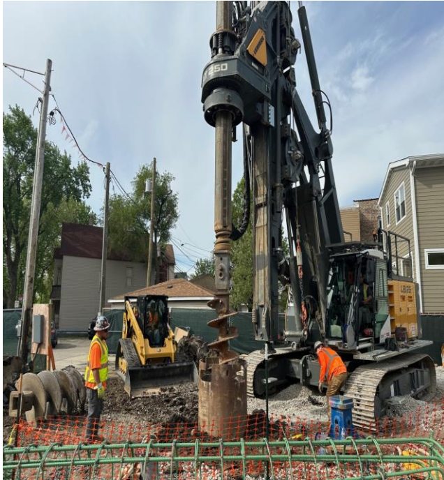
Caisson Installation at Barry
