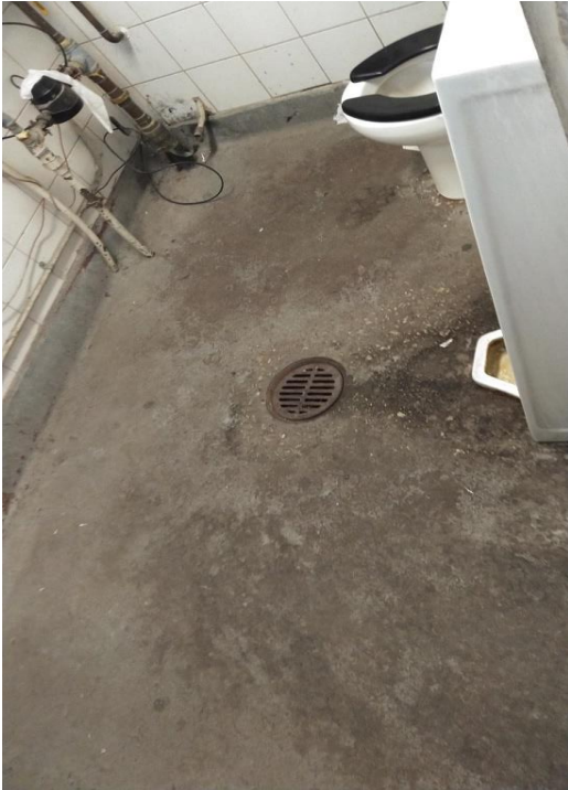
Central & Harrison – Scarify concrete floor and finish with epoxy finish
