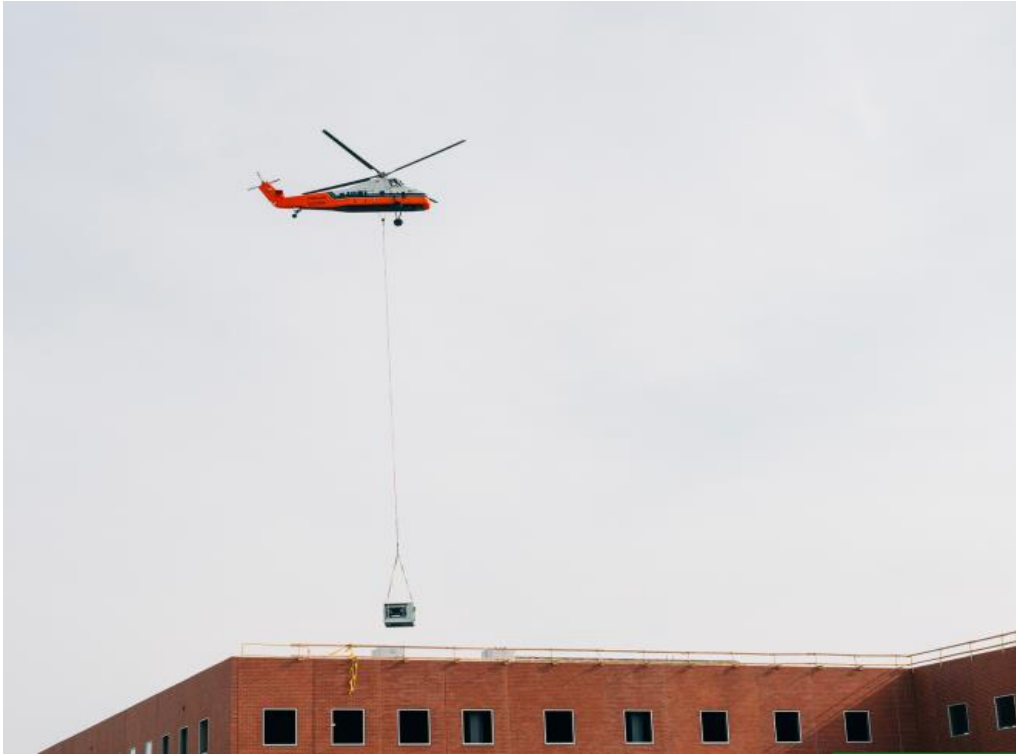
Helicopter Lift for RTU Equipment
