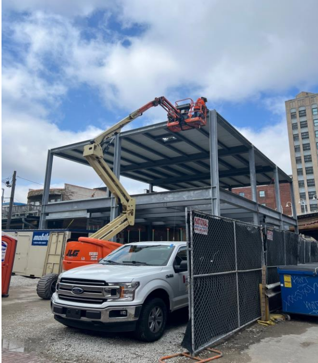
Completed Steel Erection, Roof and Plumbing Installation at Damen
