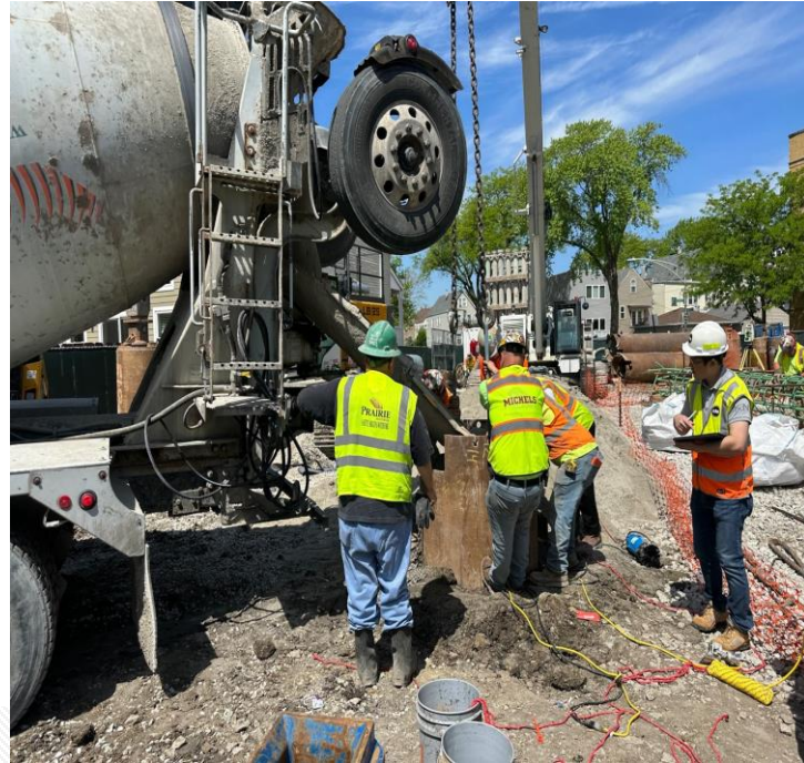
Caisson Installation at Barry
