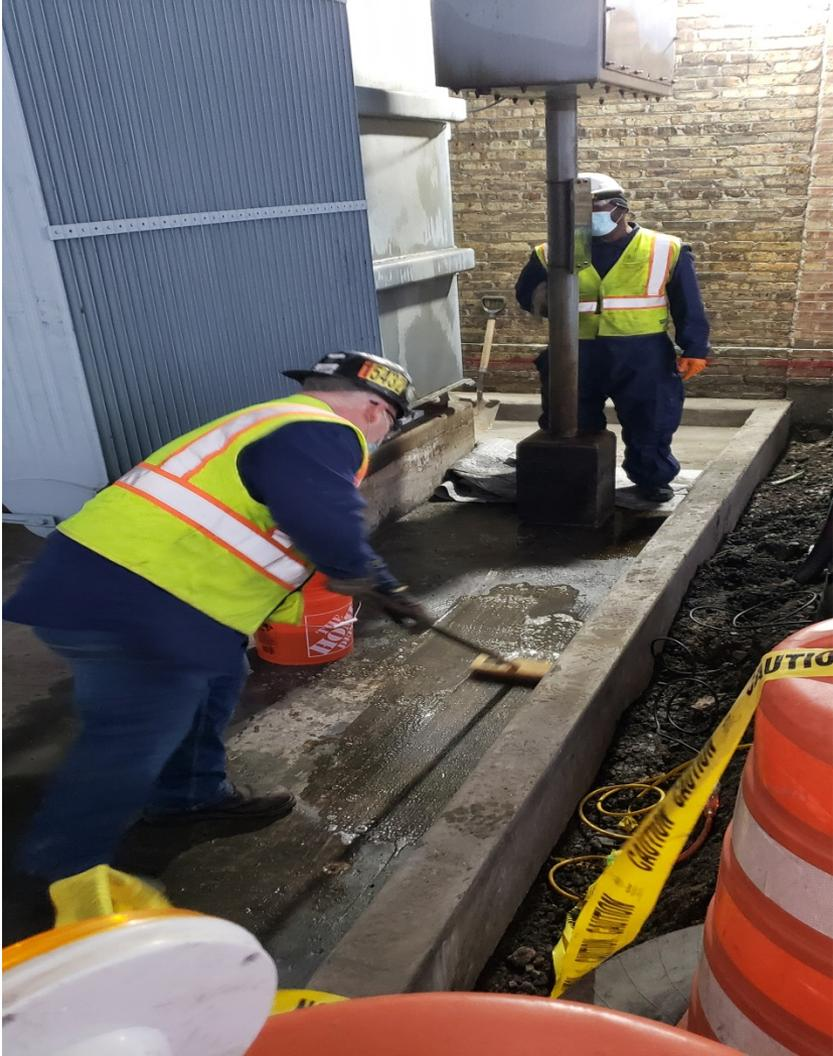
**Cleaning Concrete Pad and Conduit at Franklin Substation**
