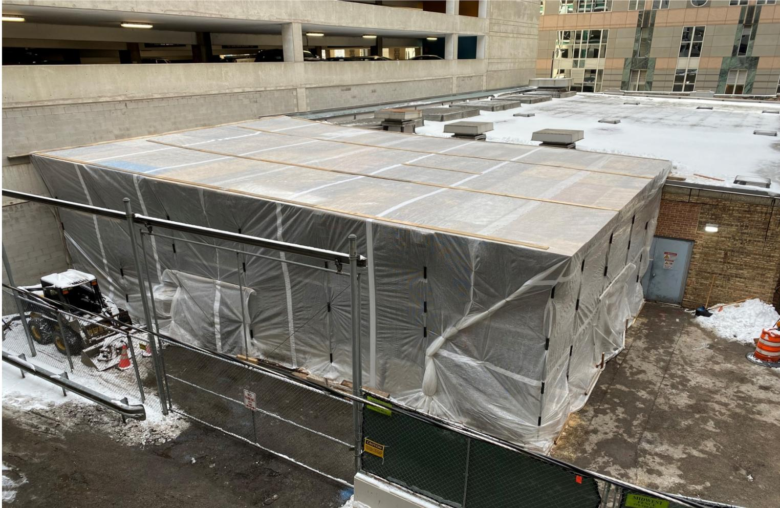
**Completed a Temporary Enclosure Around All Transformers at Franklin Substation**
