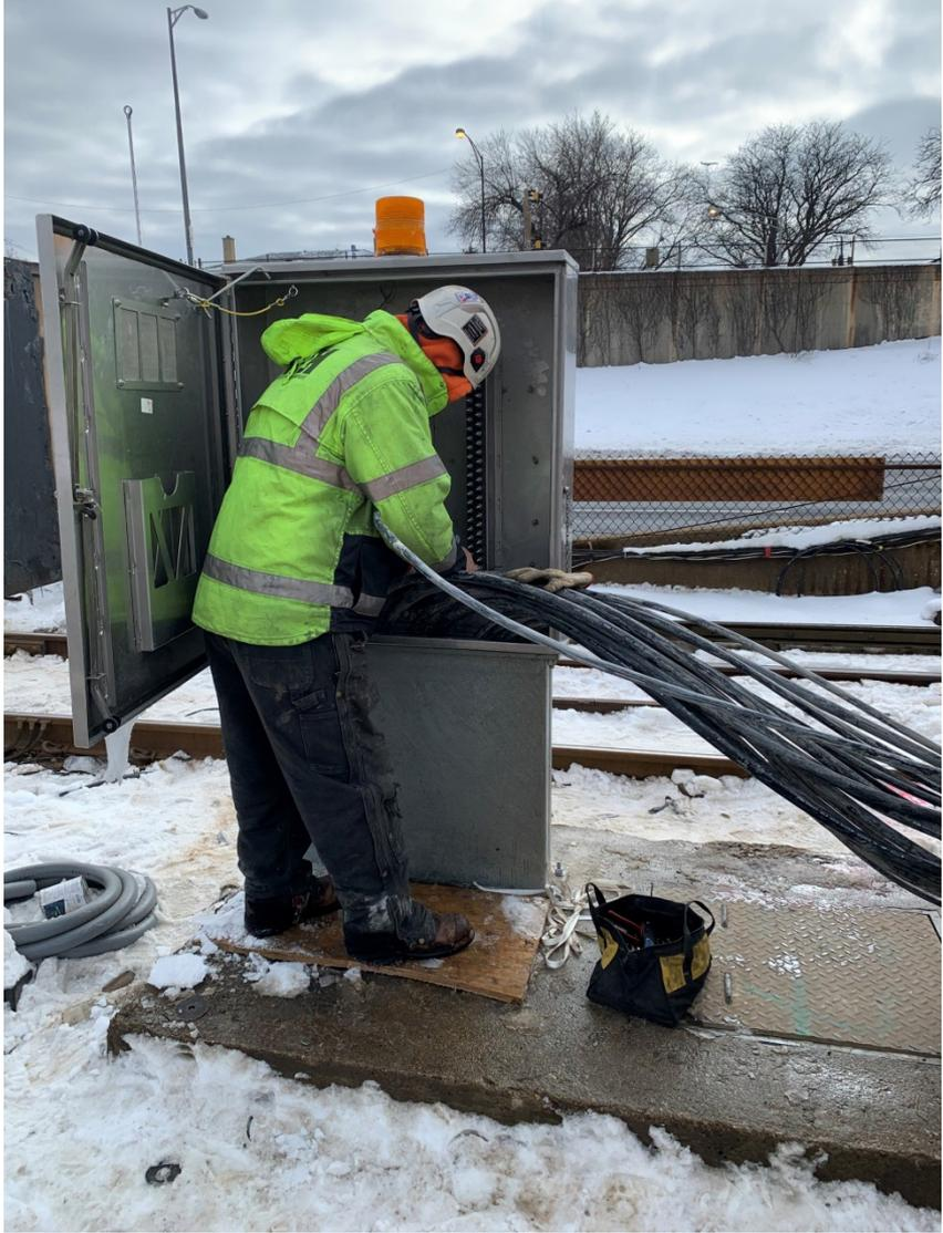
**Junction Box Wiring at Harlem Interlocking**
