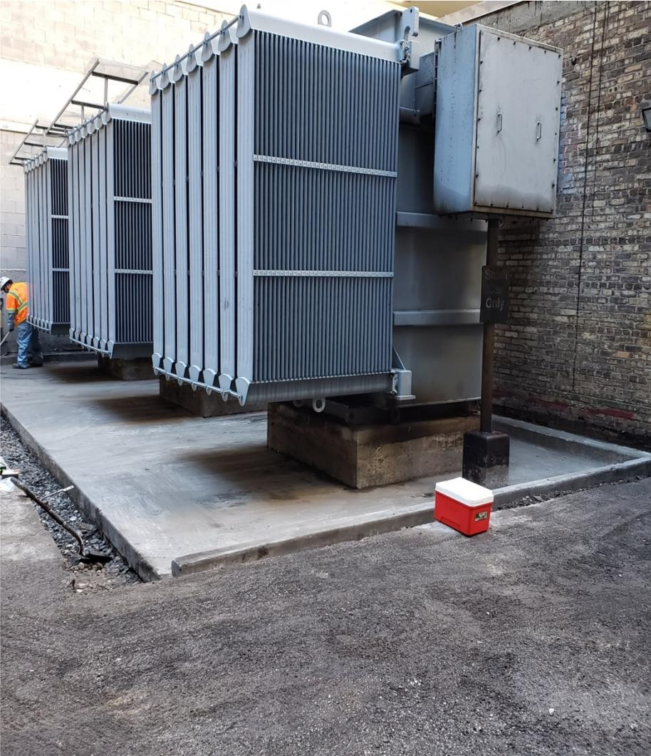
**Excavating Soil & Cleaning Existing Concrete Pad at Franklin Substation**
