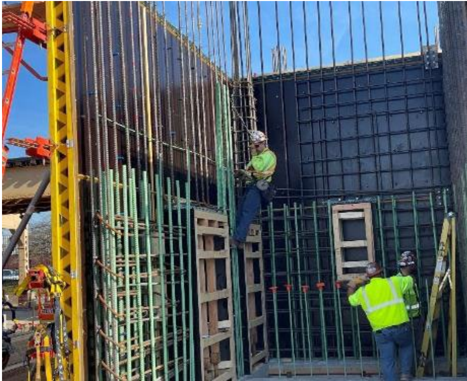
Damen Station Ironworkers installing Reinforcement Core Tower Wall
