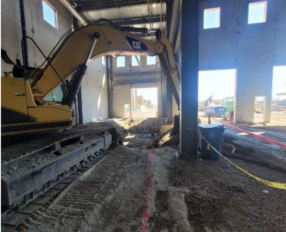
Concord – Wash Pit Excavation
