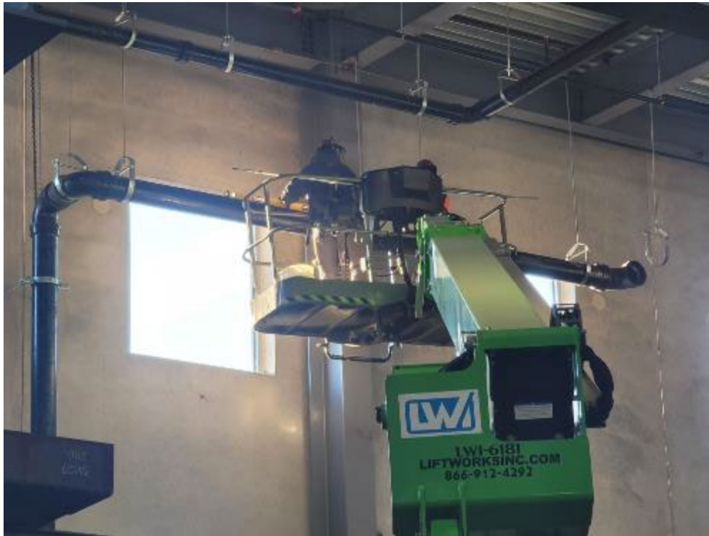
CAP - Installing Roof Drains
