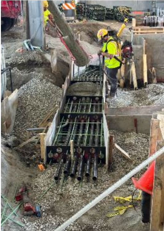
Aldridge – Pouring Duct Banks
