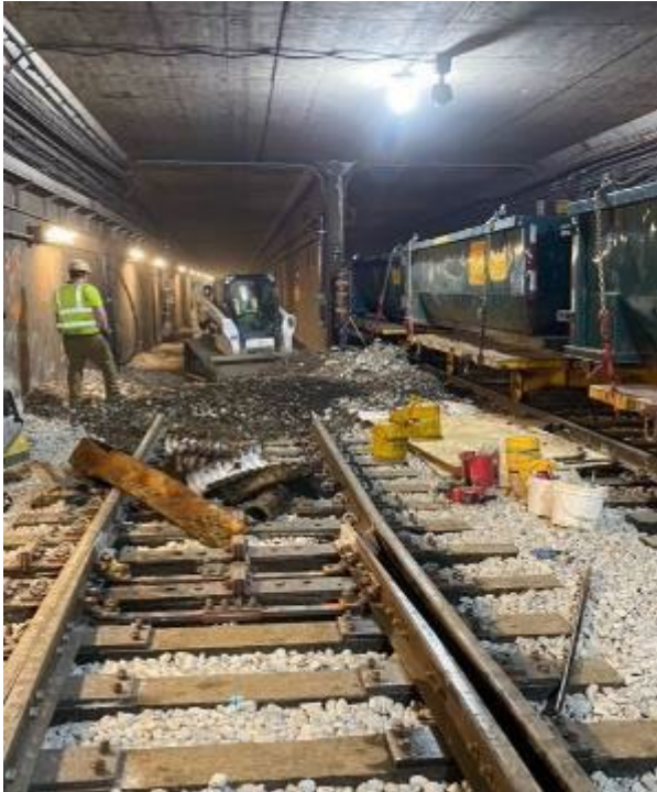
Old NB track, ballast and pre-cast walkway removal at Belmont
