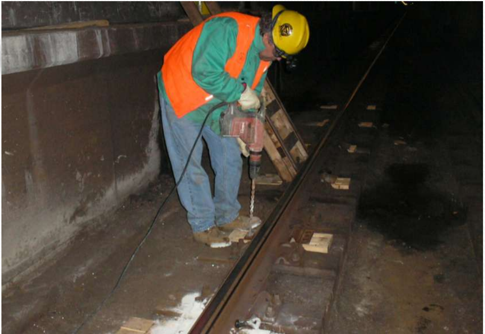
Dearborn Subway Track Work
