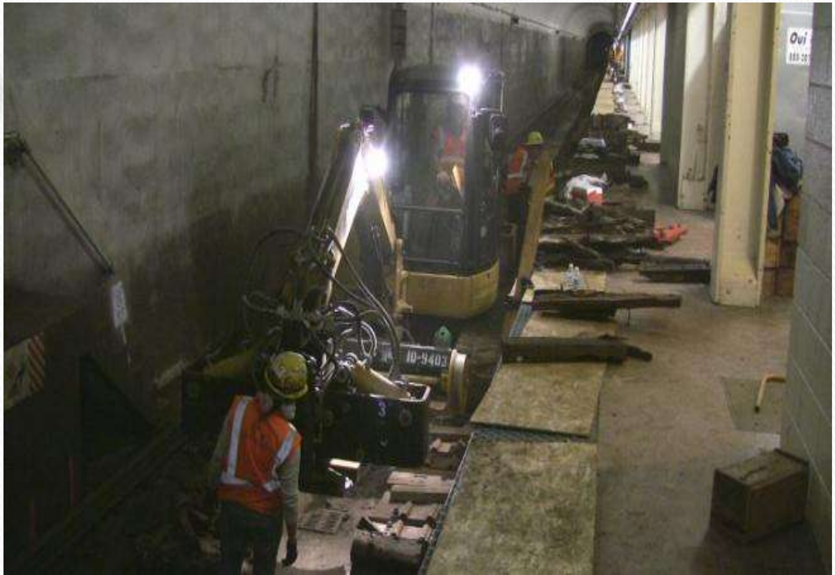
Dearborn Subway Tie Demolition
