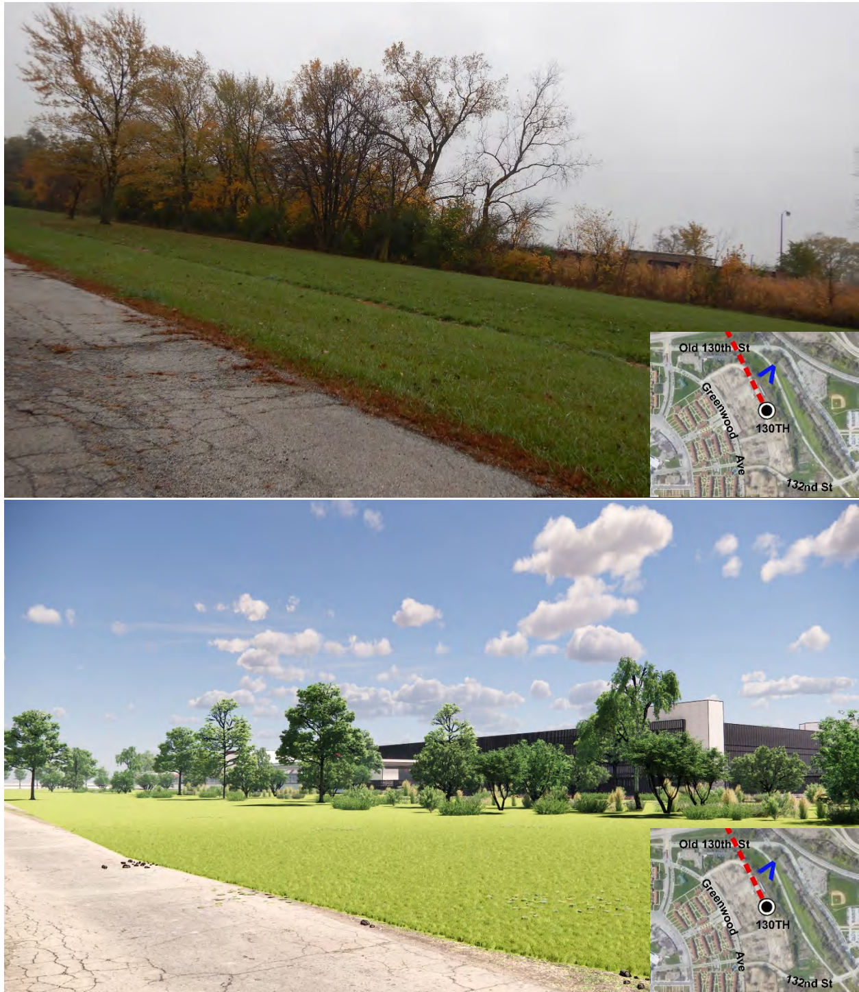
Photograph 3-3: Photo of Existing Conditions and Photo Simulation of the 130th Street Station Facing Southwest from Beaubien Woods Forest Preserve
