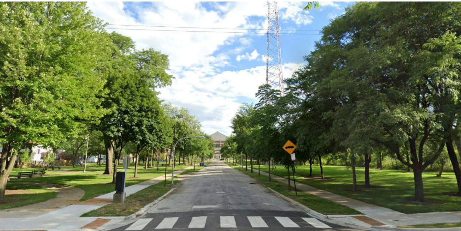
Figure 3-11: Block Park and Harvard Avenue looking toward the historic Roseland Pumping Station
