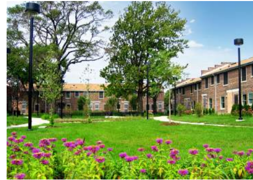
Figure 3-64: Altgeld Gardens Rowhouses Source: Chicago Housing Authority
