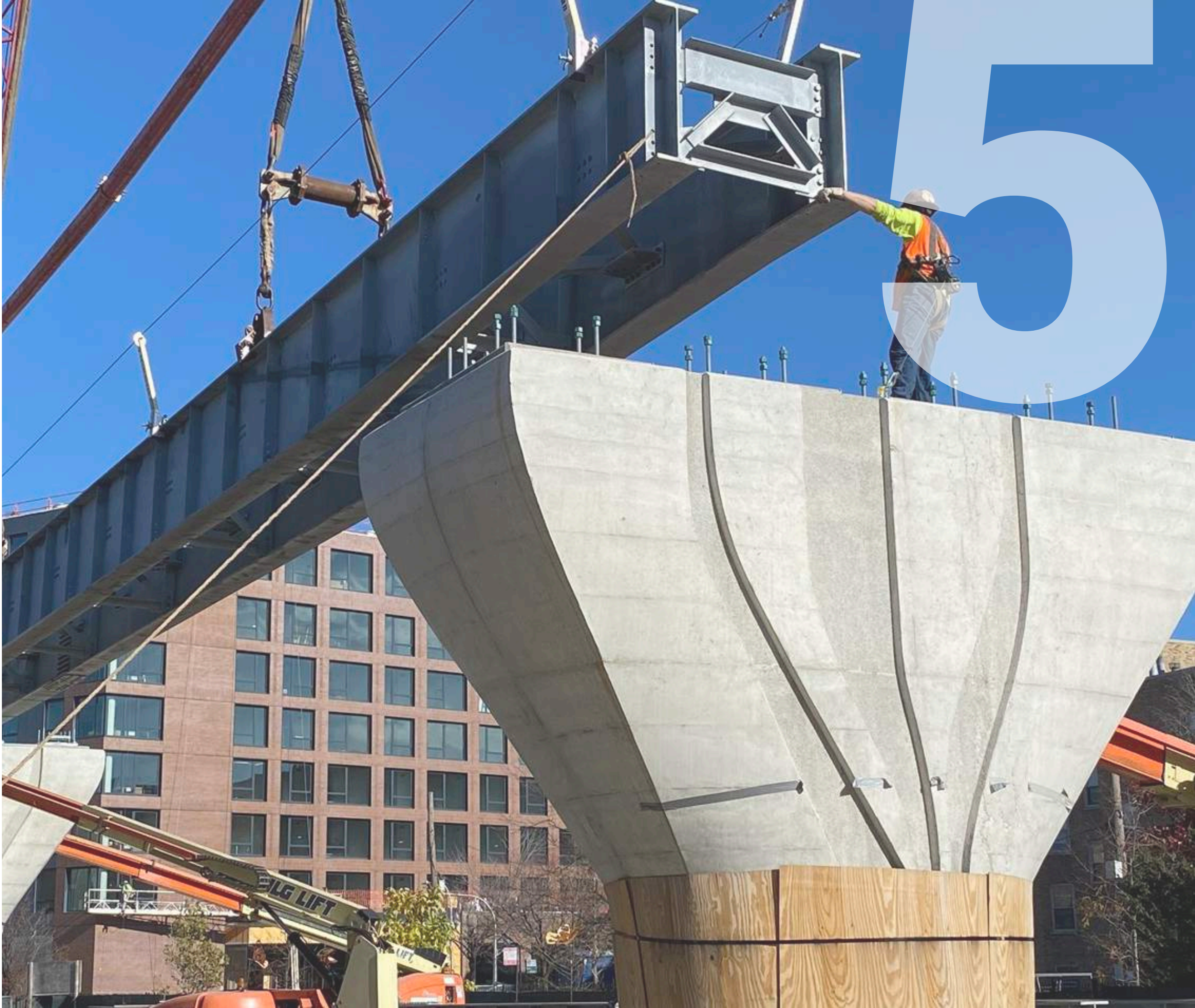
Figure 6-1: CTA Red Purple Modernization, Phase One Brown Line Bypass Construction
