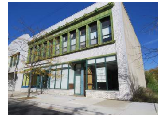
Figure 3-43: Renovated Roseland Theatre Building
