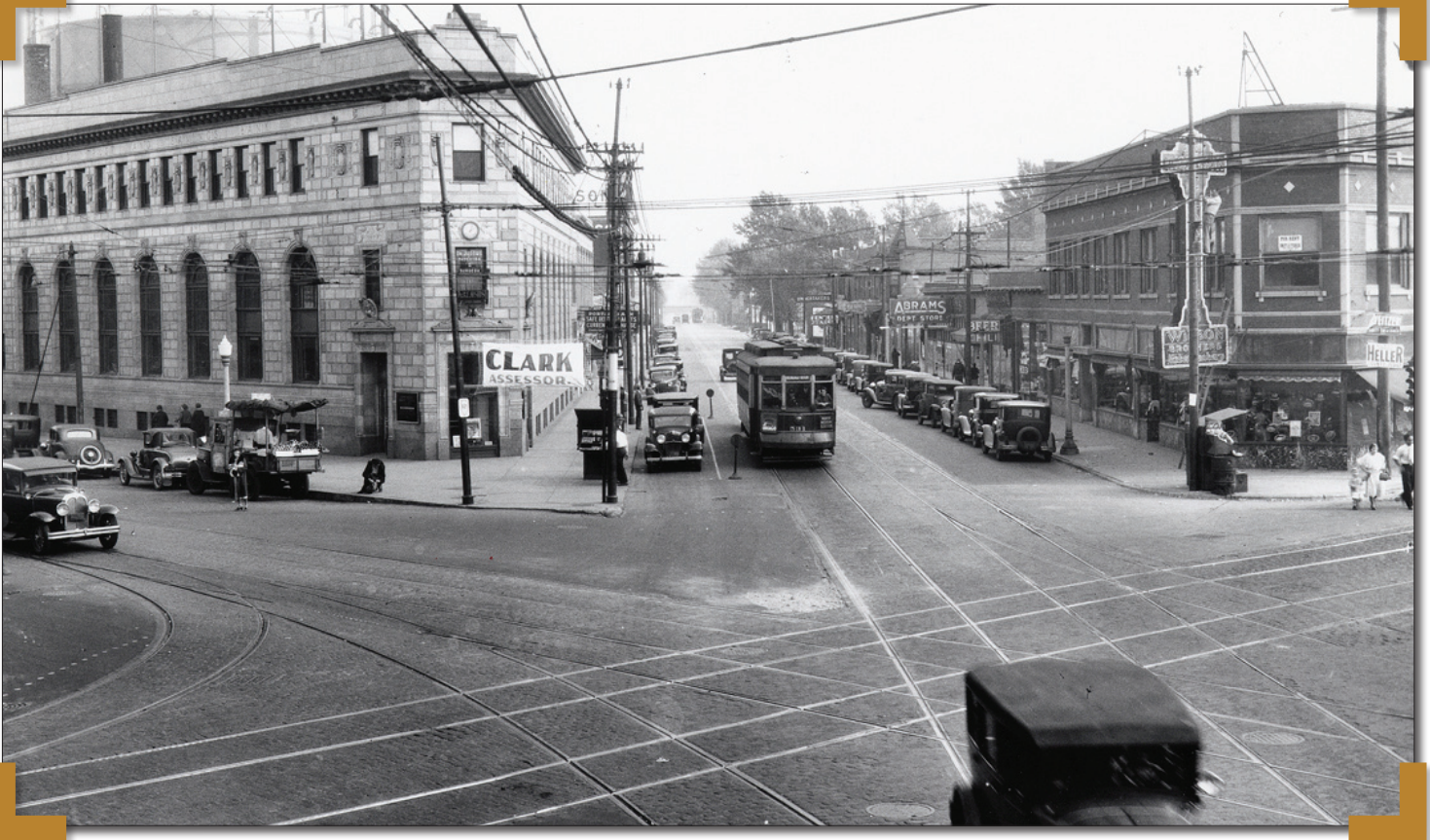
A serene view in 1934 looking southeast along Milwaukee Avenue at Irving Park/Cicero/Milwaukee. Known as "Six Corners," this intersection saw the meeting of three major streetcar lines. A northbound Chicago Surface Lines (a CTA predecessor) streetcar built by the Pullman Company in 1908 is on its way to the terminal at Milwaukee/Imlay.
