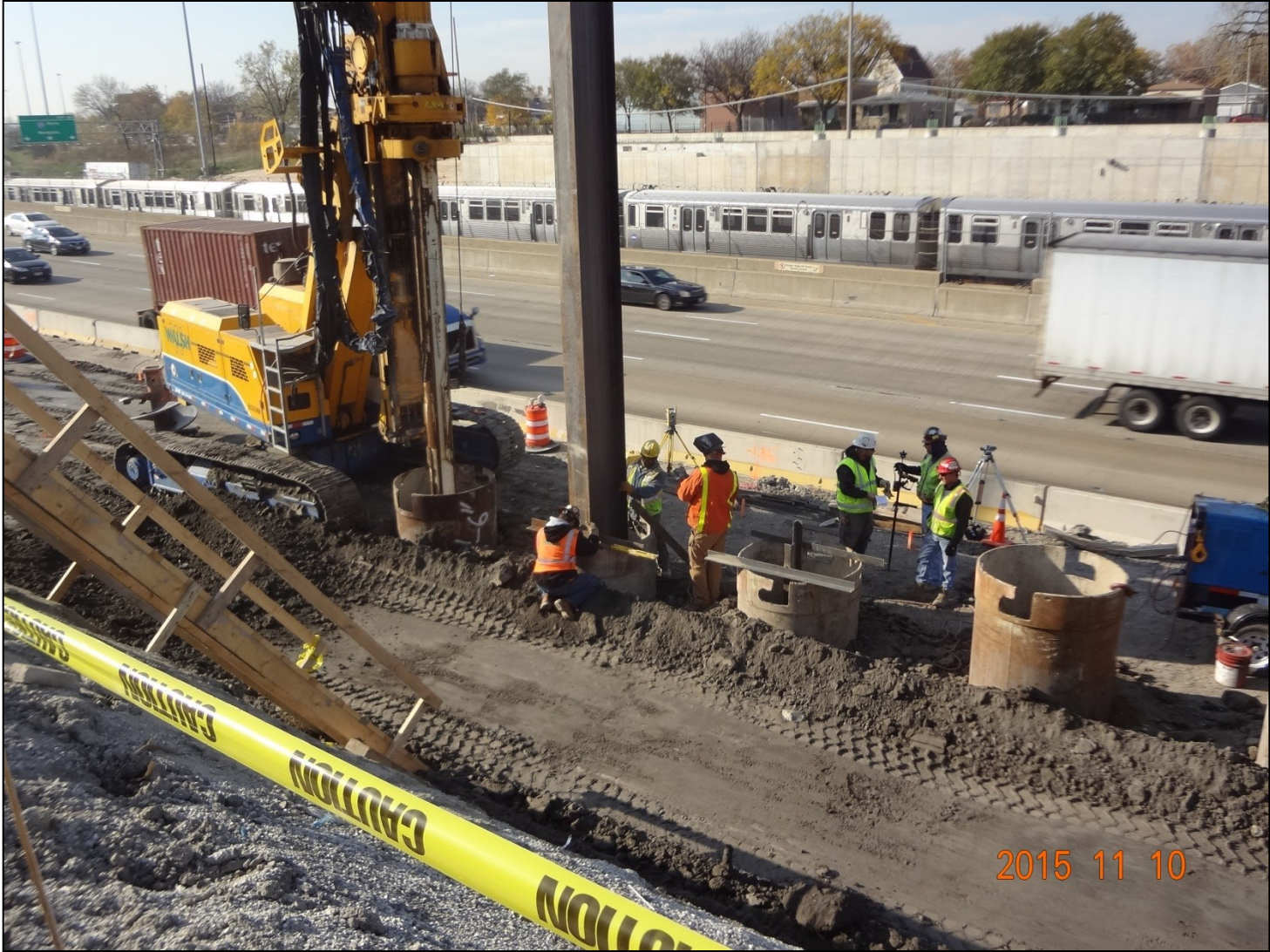
AP2: Backline SOE Installation at Wall 4
