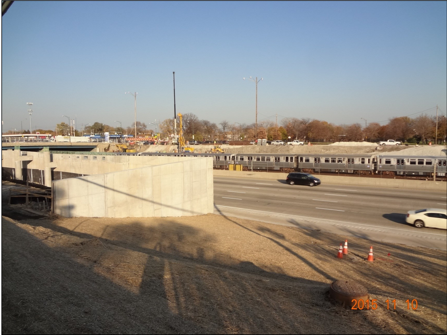
AP2: Final Seeding at Wall 1
