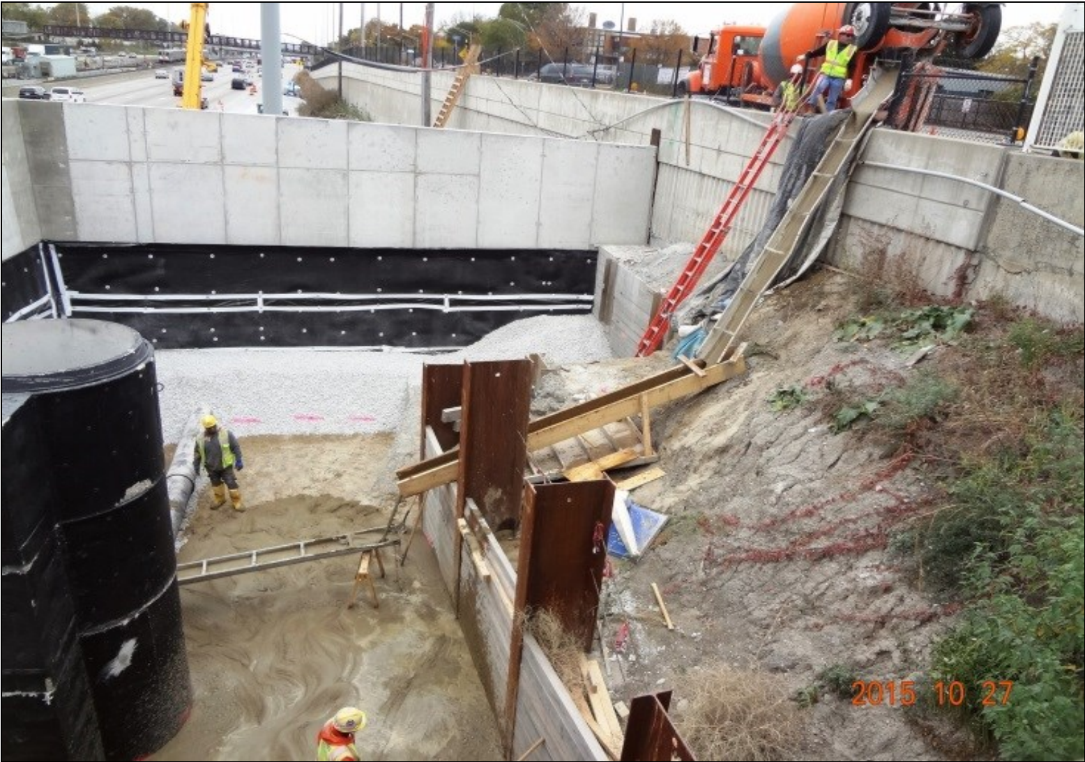
AP2: Backfill Work at Wall 6
