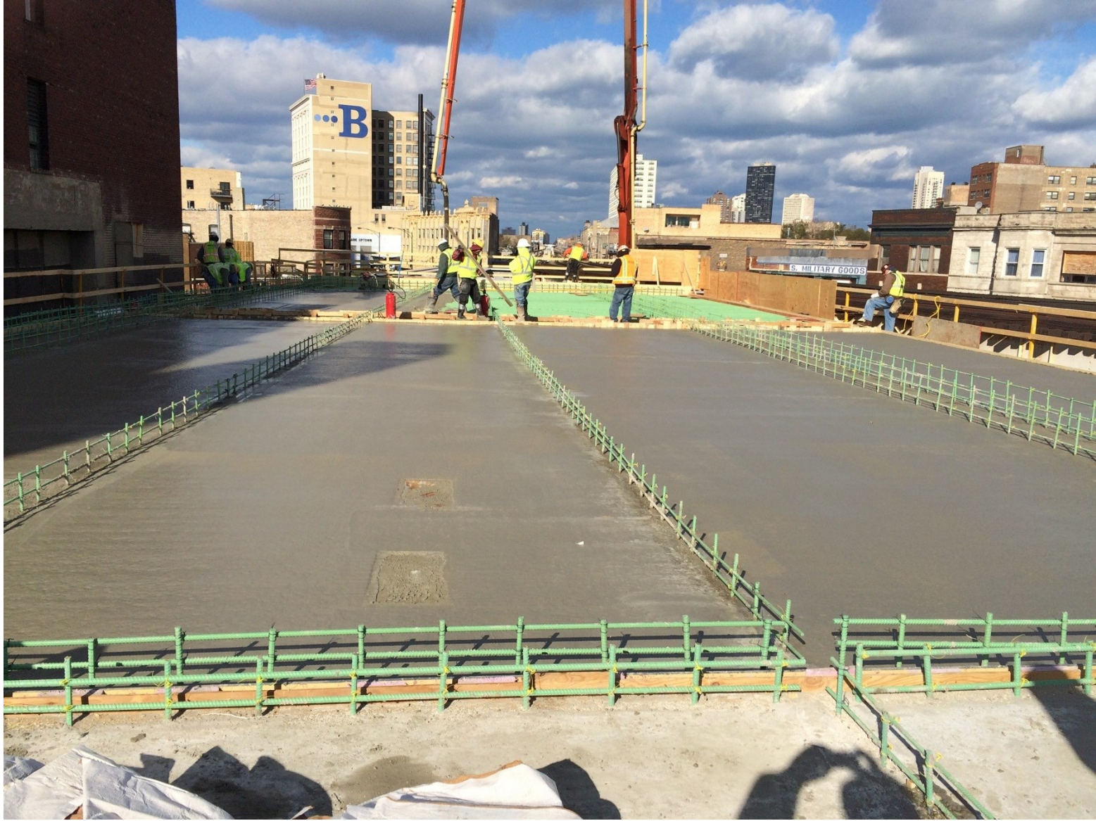
New concrete structural deck
