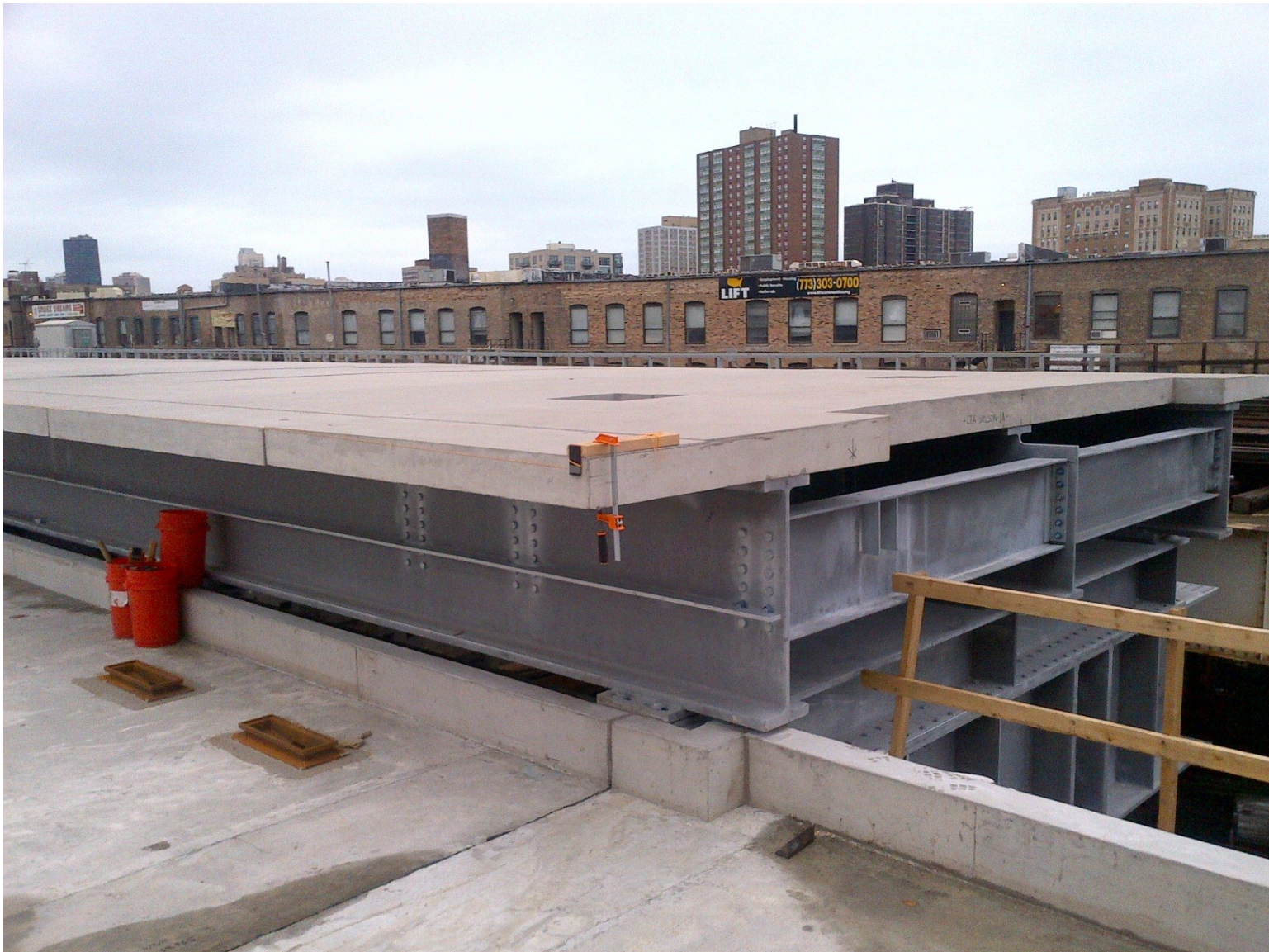
New concrete precast platform installation
