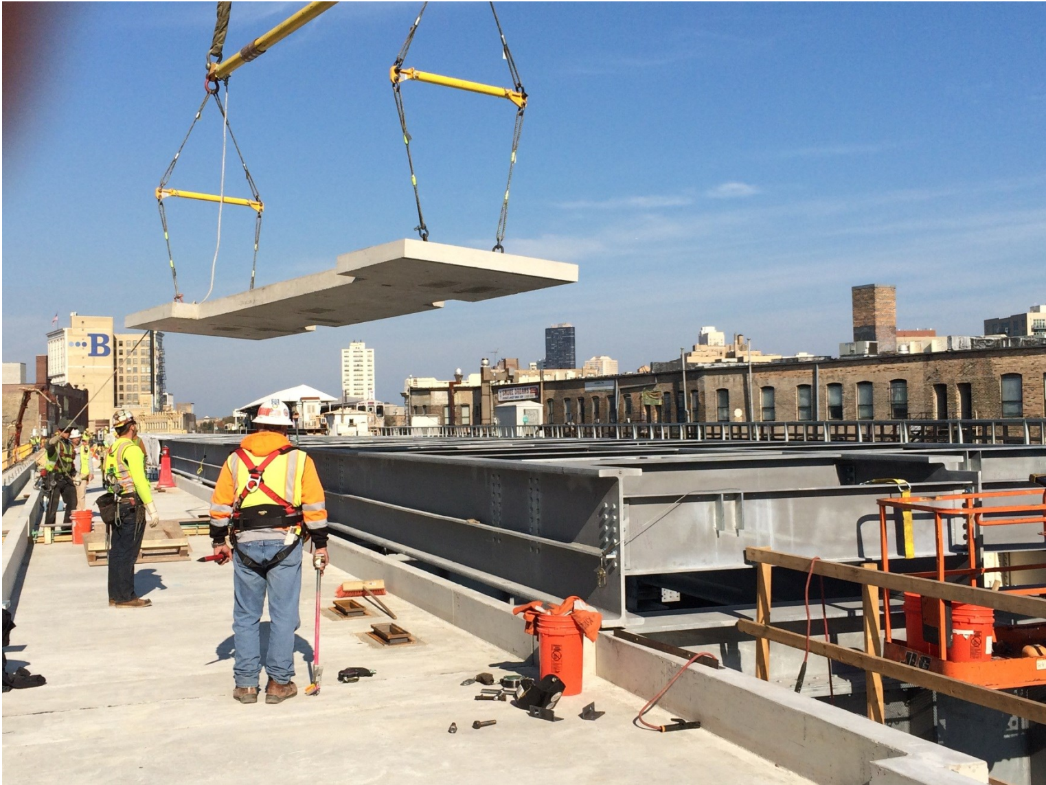
New concrete precast platform installation
