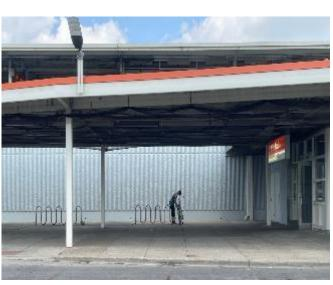
**35<sup>th</sup>/Archer –** Paint all columns and under canopy. Re-attach all pigeon deterrent netting.
