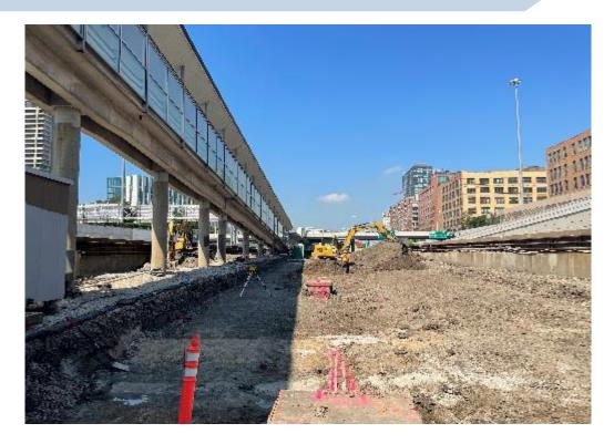
Mass Excavation & Grading by UIC-Halsted Station
