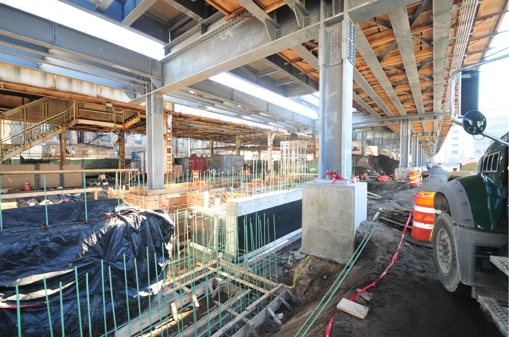
New Wilson Station Foundations
