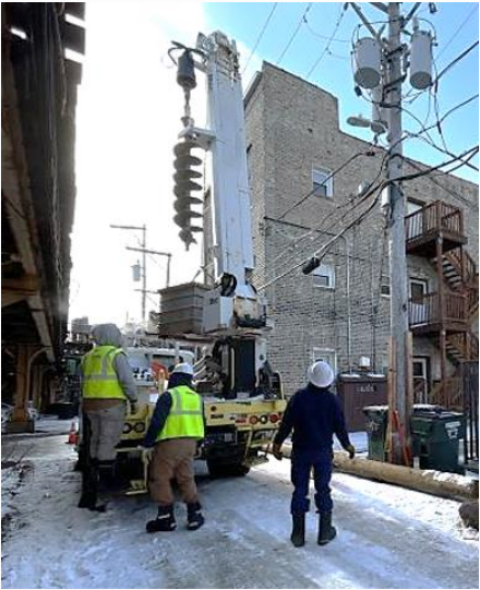
Light pole digging/setting truck
