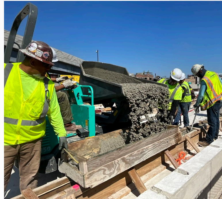
Concrete pour, RPM Phase One Project
