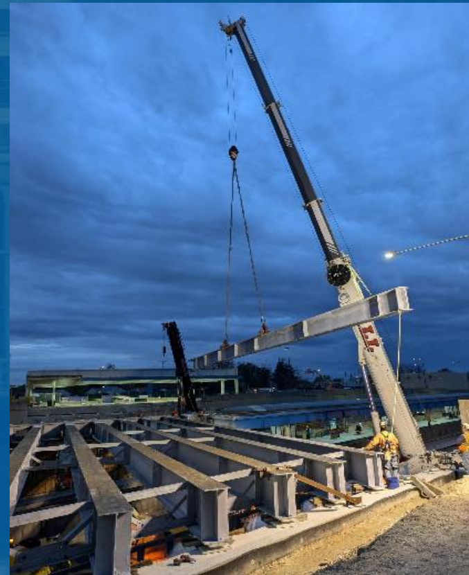
Bridge Beam Installation
