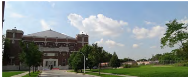
East Option Elevated Track Structure adjacent to the Roseland Pumping Station, Facing South on Harvard Avenue
