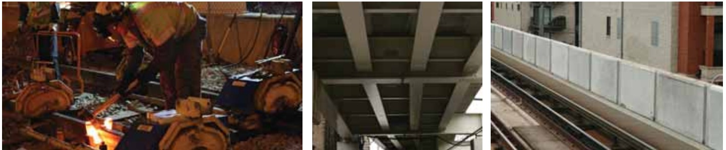
Closed Deck, Welded Rail with Noise Barriers
