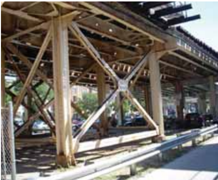
CTA Elevated Track Structure
